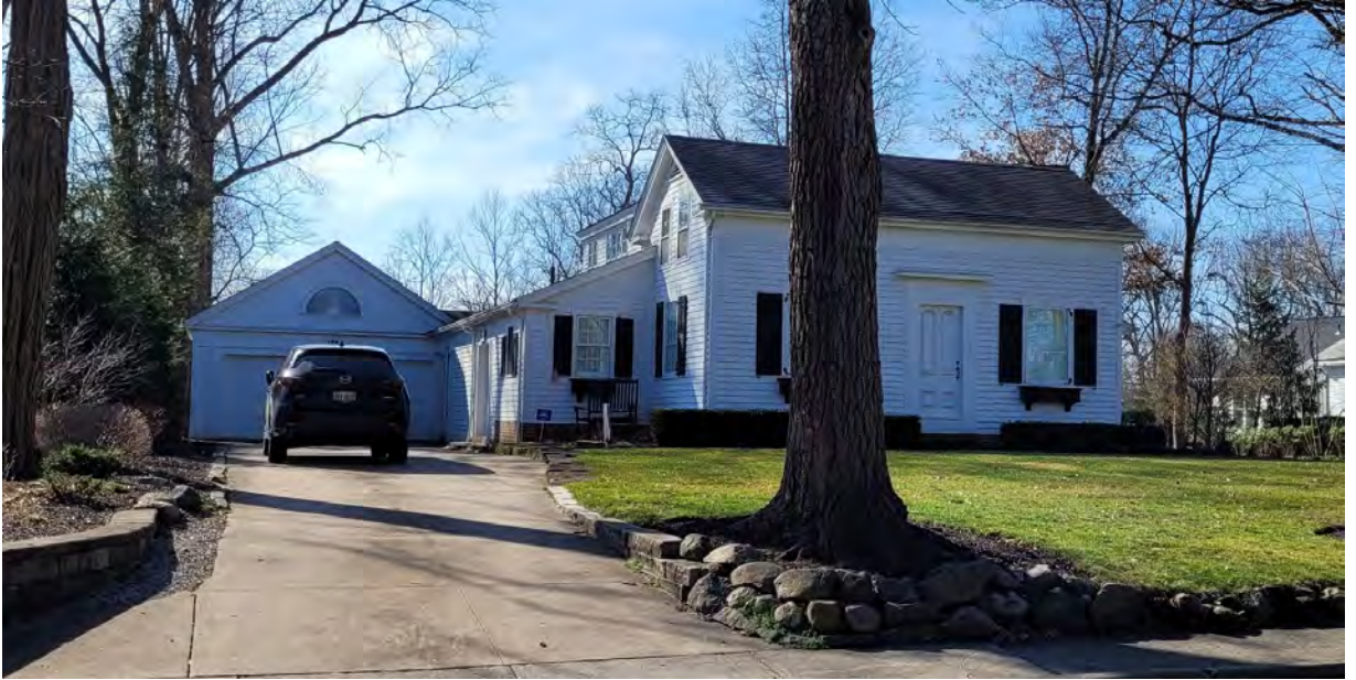
Image 13: House while standing across the street.
