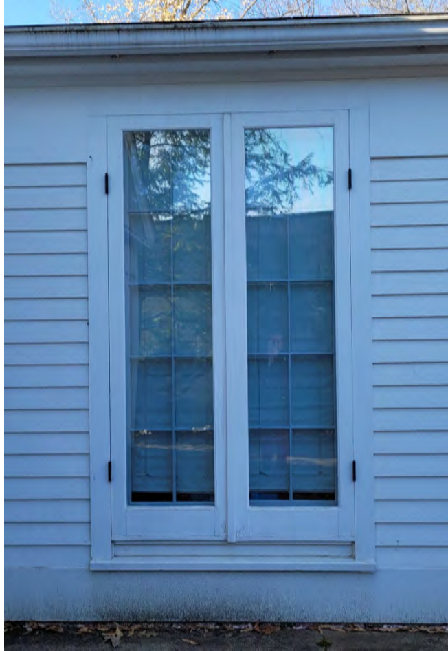
Image 16: Side (east) elevation wood door to be removed.
