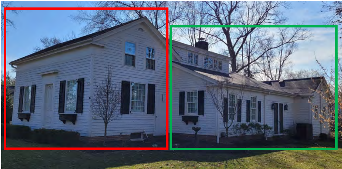
Image 12: Front (north) and side (west) elevations. The red box indicates the original house that dates to c1854. The green box indicates the addition that dates to 1997.
