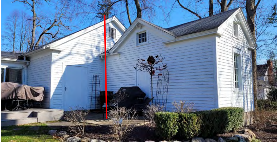
Image 11: Side (west) and rear (south) elevations. The portion to the left of the red line is the 1985 addition and the portion to the right of the red line is the garage that reportedly dates to 1936.
