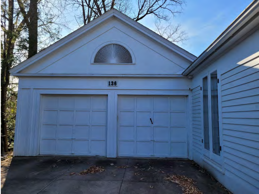
Image 7: Front (north) elevation of the attached 1985 garage.
