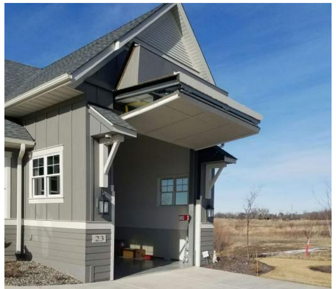
With no loss of headroom and some to spare, the 16' tall clear opening is big enough for even the largest RV to drive in and out.
