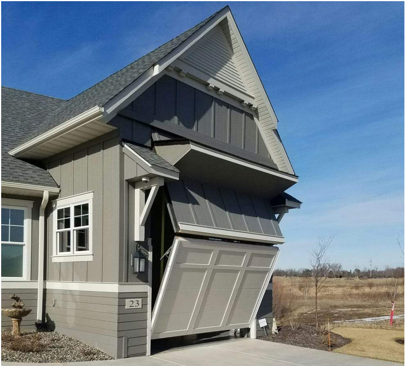
When partially open you can easily see where the door bends in the middle. An eave was placed on the upper portion of the bifold door to match the rooflines of the home.
