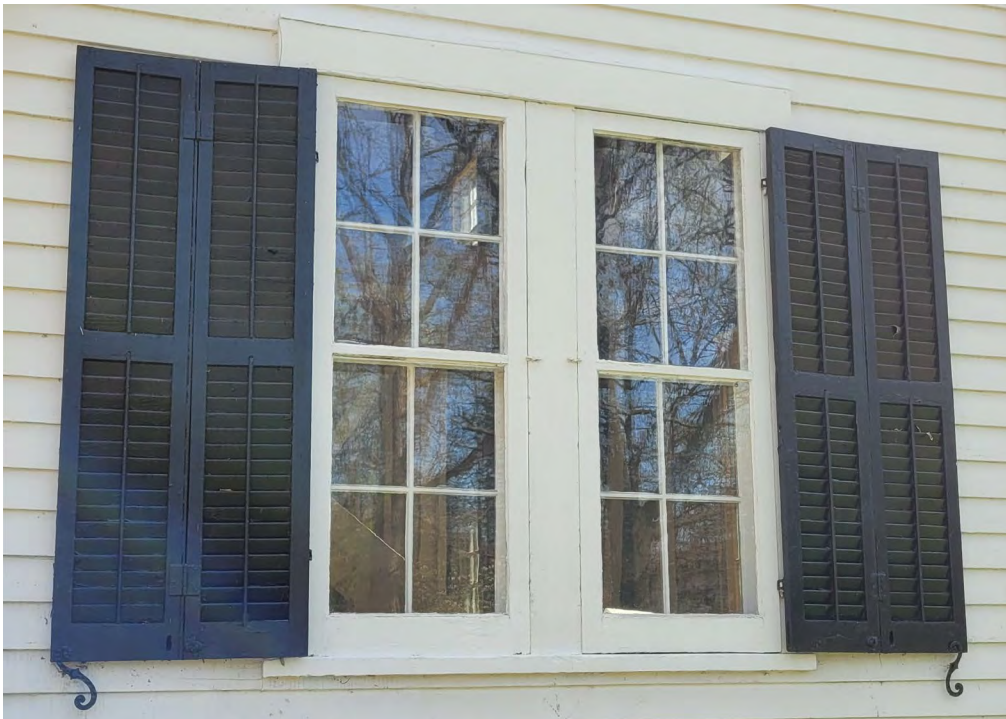
Image 9: Detail of front (north) historic wood paired window to be replaced.
