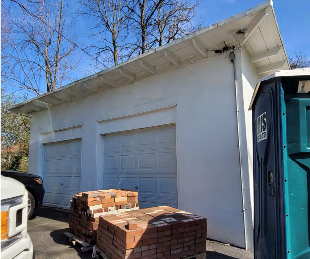
Image 12: Front (north) of garage.
