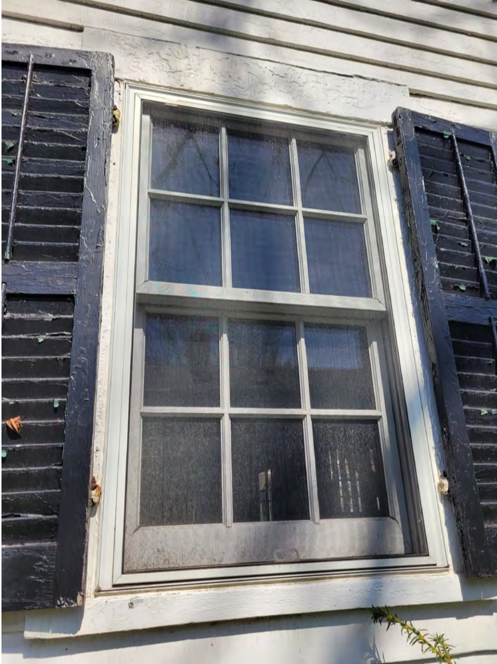
Image 10: Detail of typical vinyl replacement window to be replaced.
