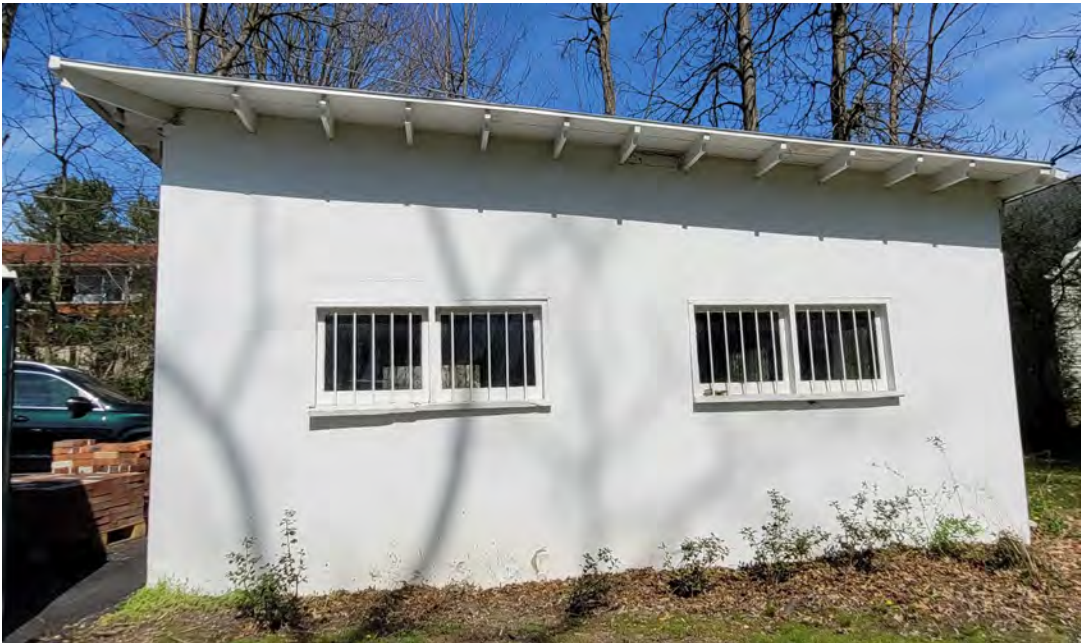
Image 13: Side (west) elevation of garage.
