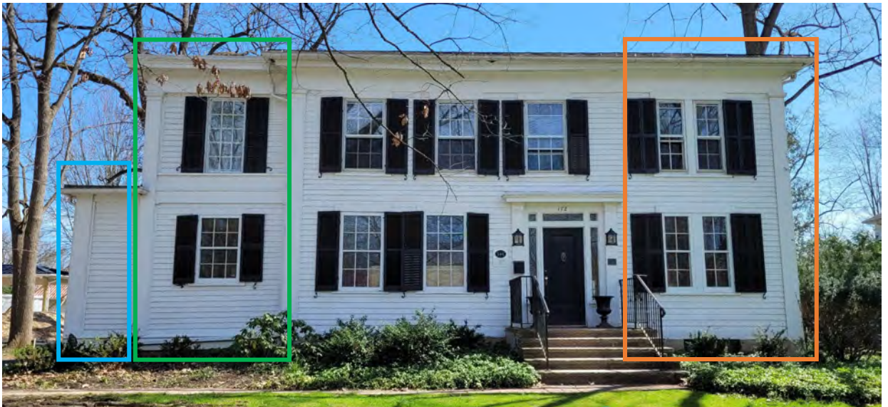
Image 3: Front (north) elevation. The orange box indicates the 1913 addition. The green box indicates the 1925 addition. The blue box indicates an addition with an unknown date.
