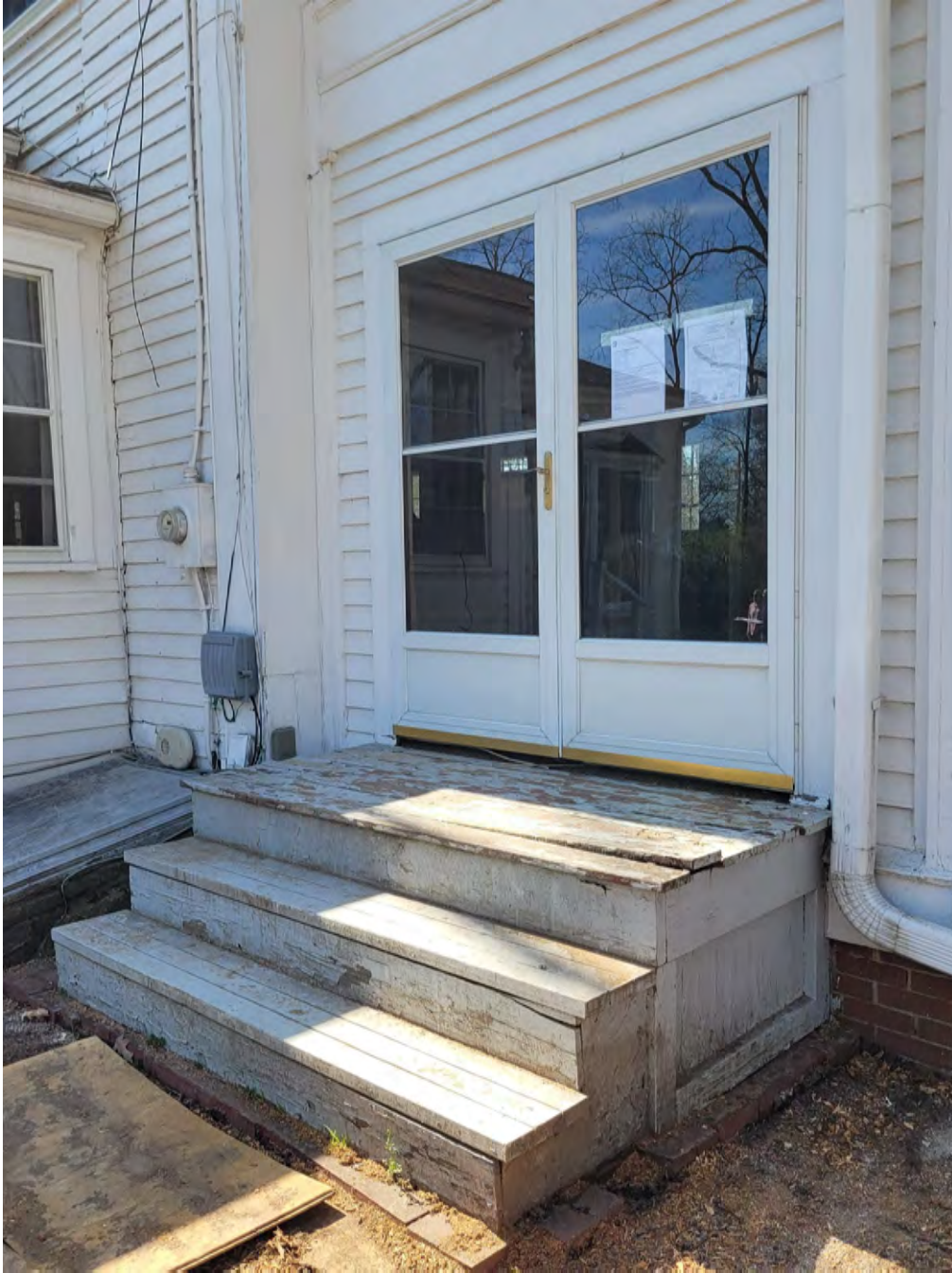
Image 11: Detail of wood staircase and replacement French doors to be removed.
