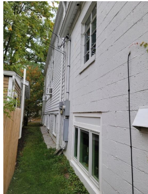
Side of building. No doors
