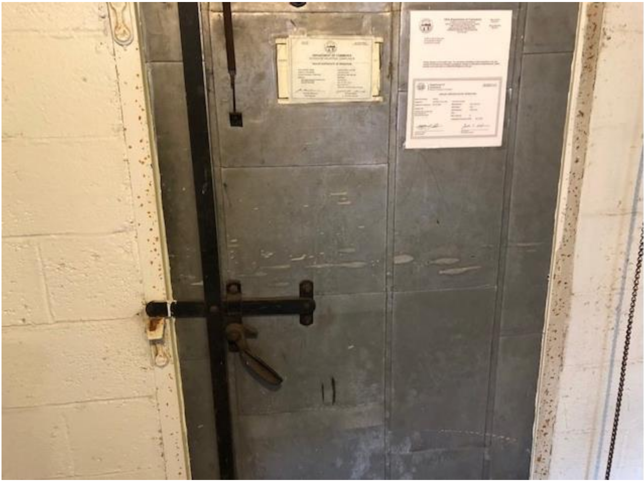
Figure 9 - possible SAFE ROOM - Boiler room
