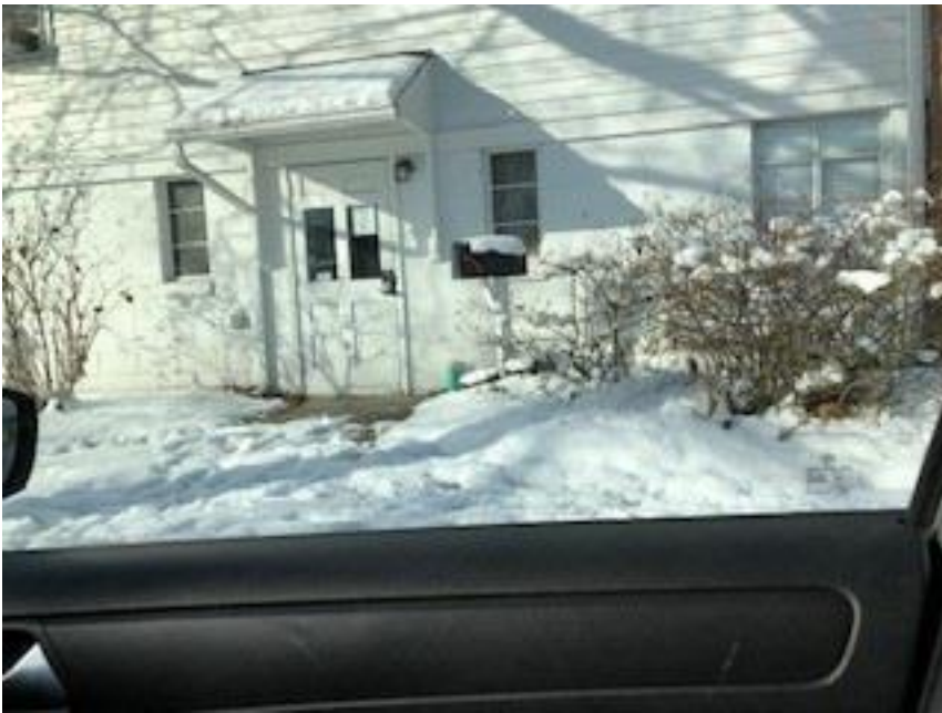
Figure 5 exterior entrance on College Street - side door
