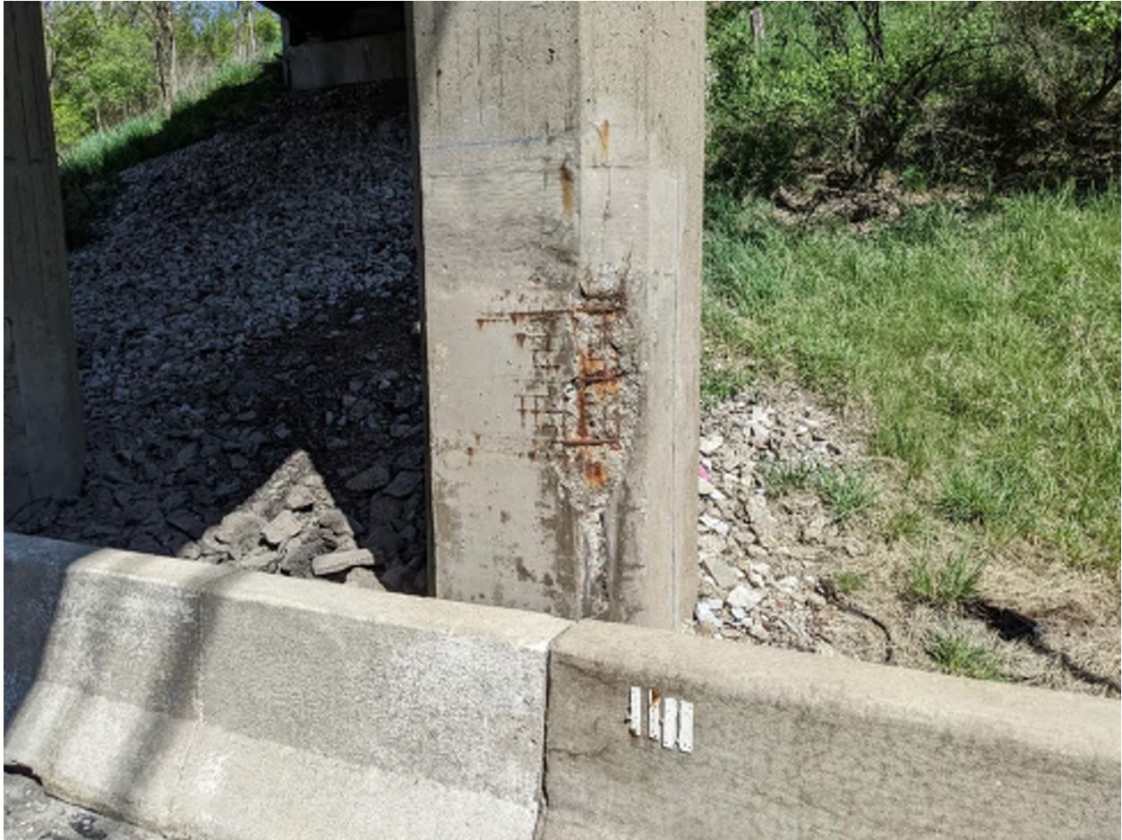
Photograph #12 - Pier 3 Column 3 Spall MP 182.1
