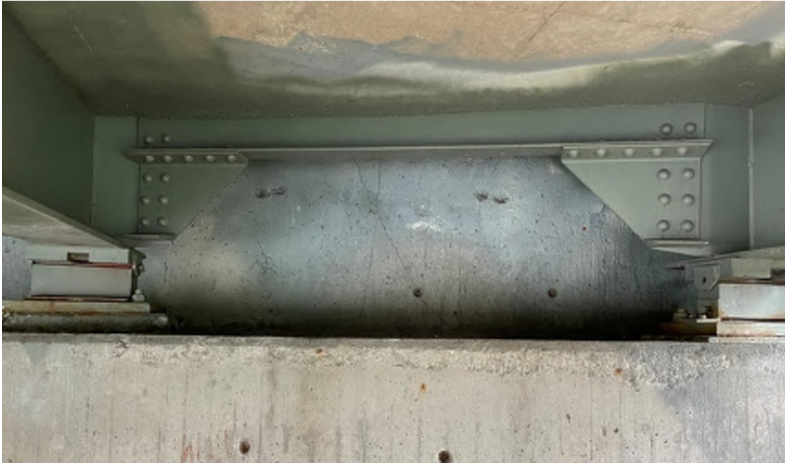
Photograph #4 - Typical End Diaphragm Condition (Main Span) MP 182.1
