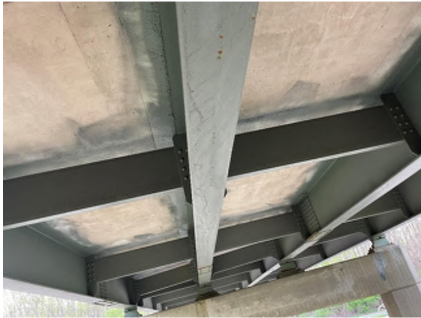
Photograph #2 - Typical Beam and Intermediate Diaphragm Condition (End Spans) MP 182.1
