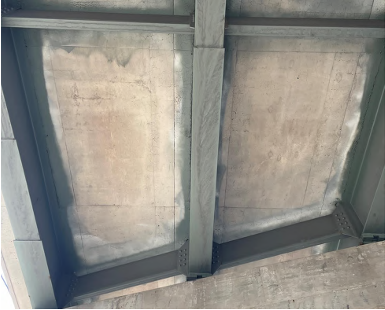
Photograph #6 - Typical Moment Plate Condition MP 182.1
