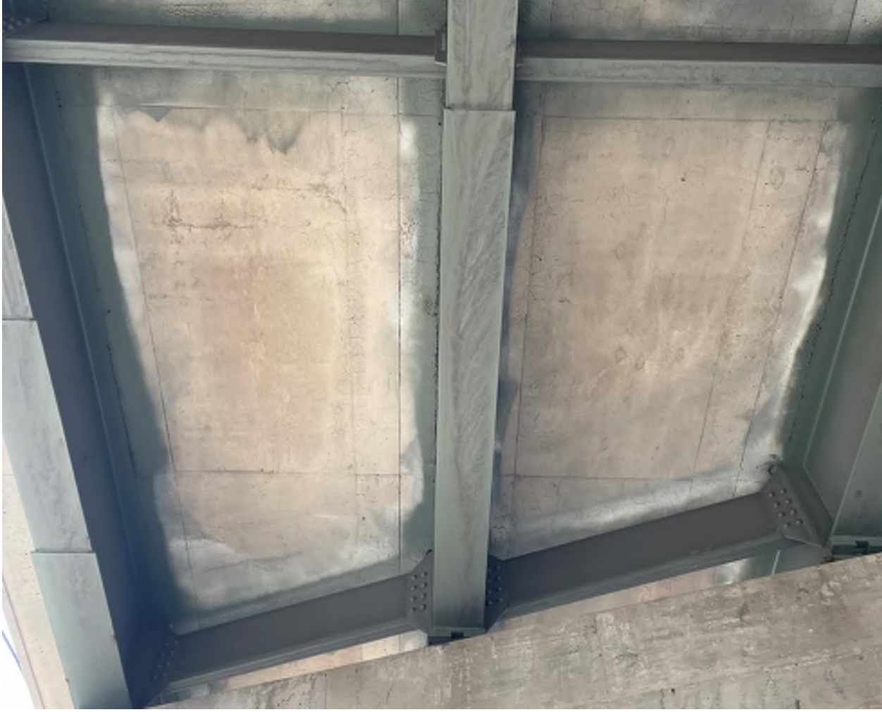
Photograph #6 - Typical Moment Plate Condition MP 182.1
