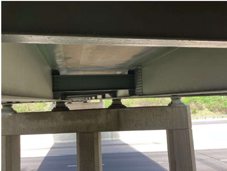
PHOTO 2 View of structure underside. No utilities were affixed.
