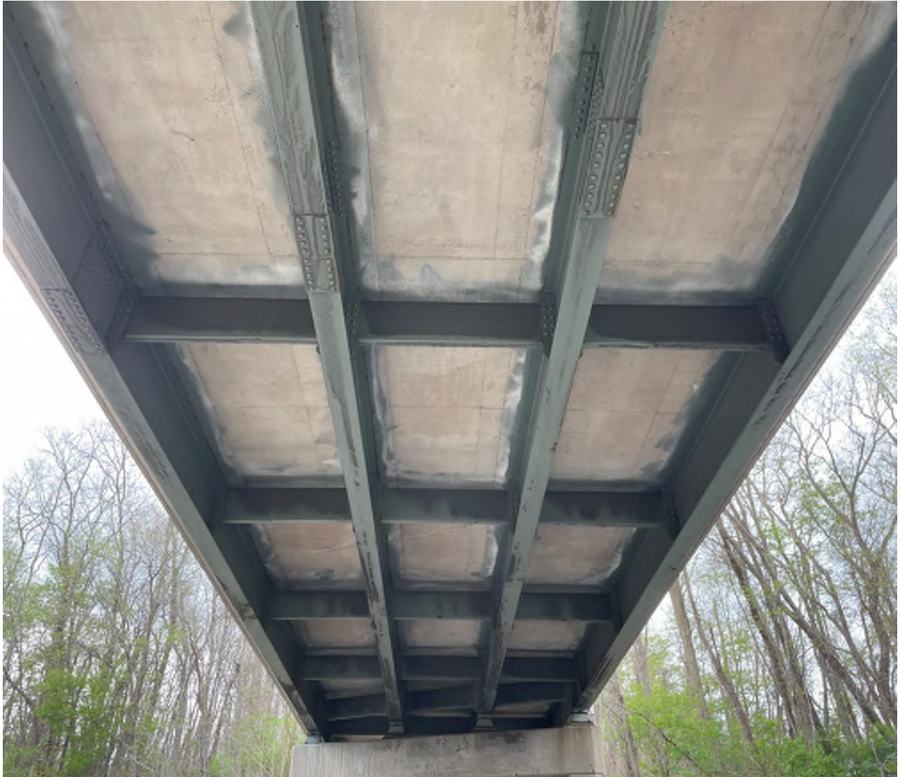
Photograph #3 - Typical Beam and Intermediate Diaphragm Condition (Main Spans) MP 182.1
