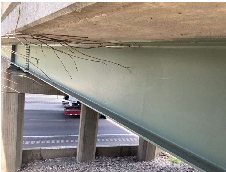
PHOTO 5 View of outer beam. Paint in good condition.
