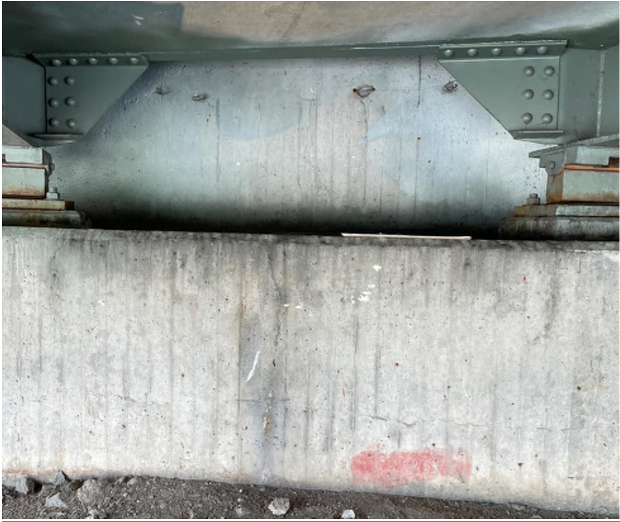
Photograph #8 - Forward (North) Abutment Vertical Crack MP 182.1
