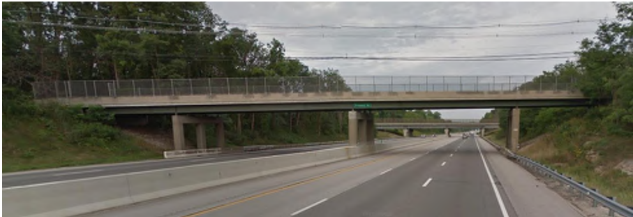
Photograph #1 - Partial Elevation of Right Fascia (looking West)
