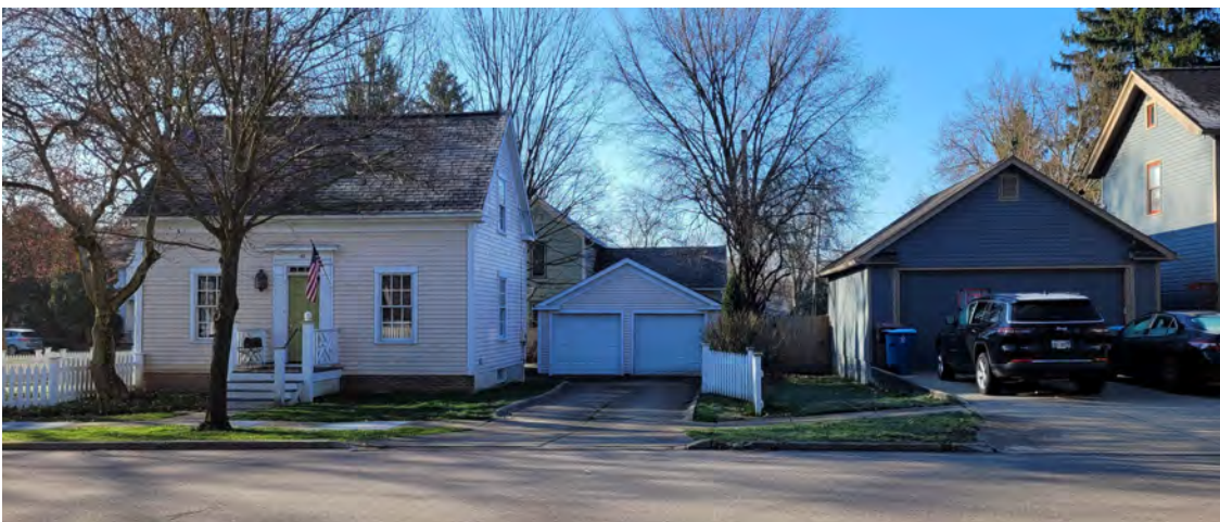
Image 12: Hudson National Register Historic District contributing houses to the southeast of 43 Church Street.
