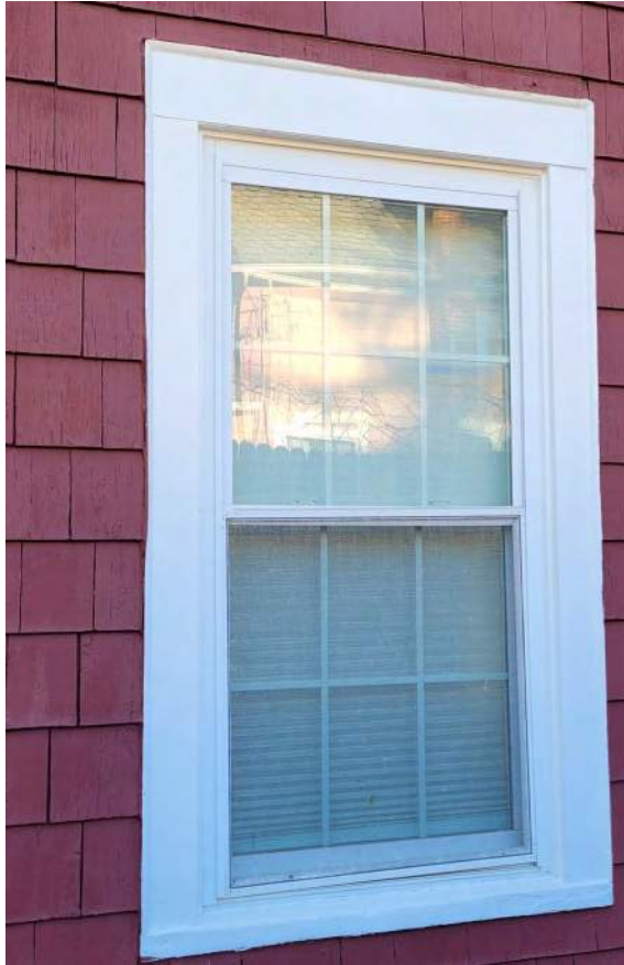
Image 8: Detail of side (west) non-historic vinyl window to be potentially reinstalled in the new one story mass on the side (west) elevation.
