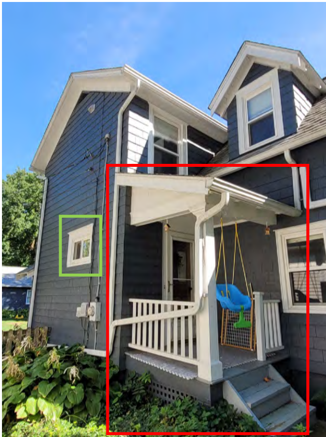
Image 8: Side (north) elevation. The red box indicates the covered side porch that appears to have been previously altered and is proposed to be enclosed. The green box indicates the window to be replaced and moved.
