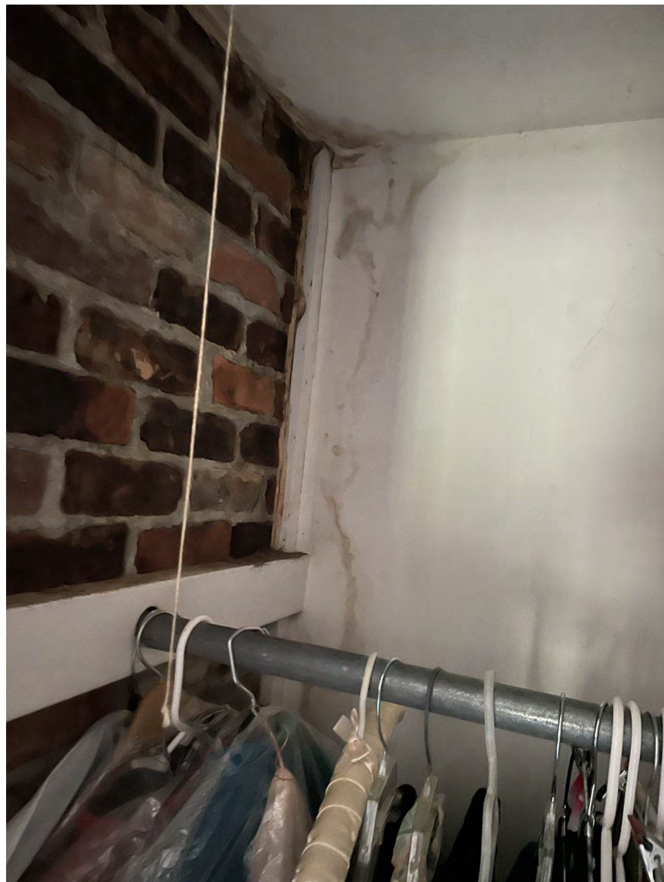
IMAGE OF THE EXISTING INTERIOR FOR REFERENCE - CLOSET
