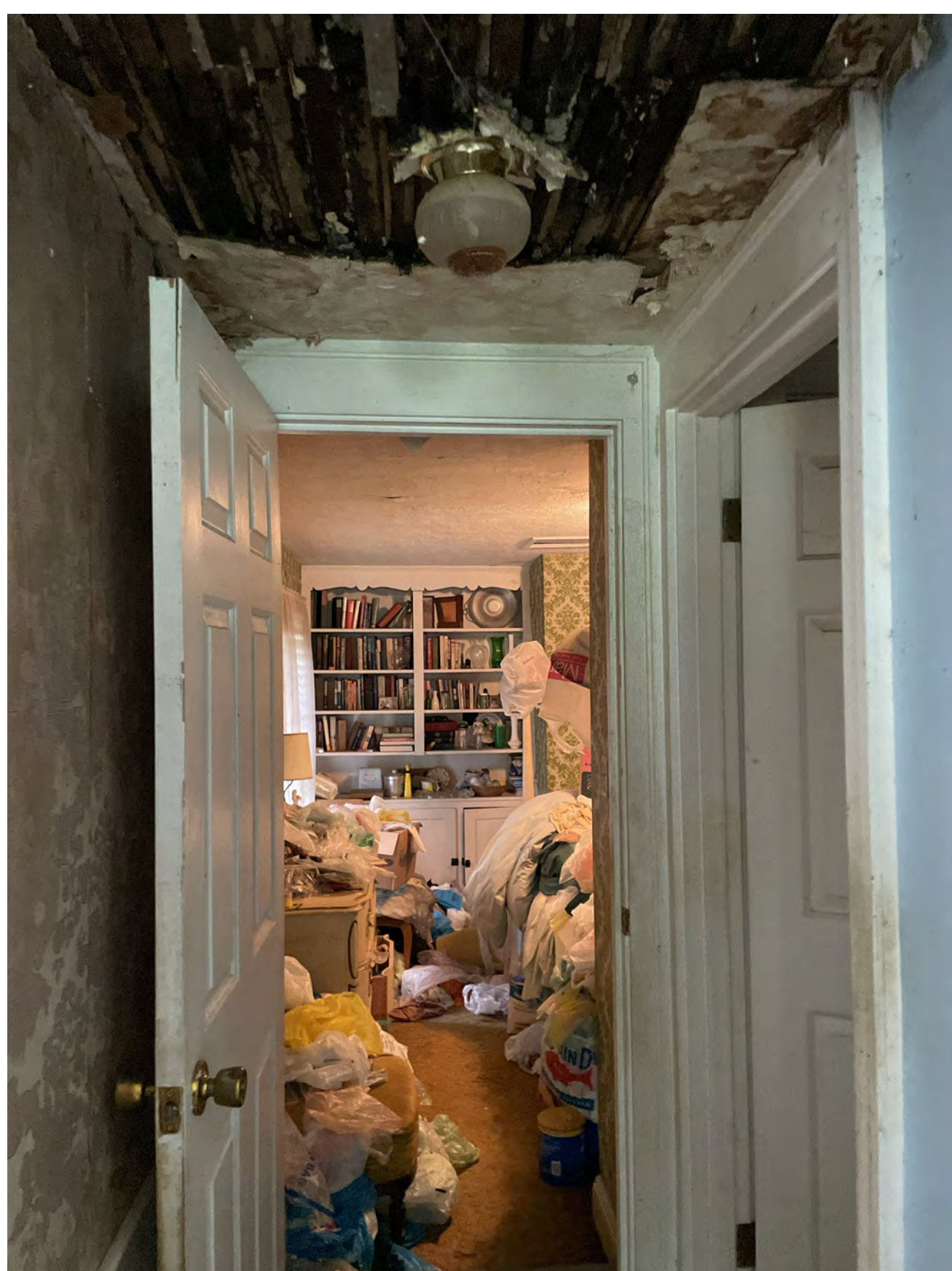
IMAGE OF THE EXISTING INTERIOR FOR REFERENCE - HALL
