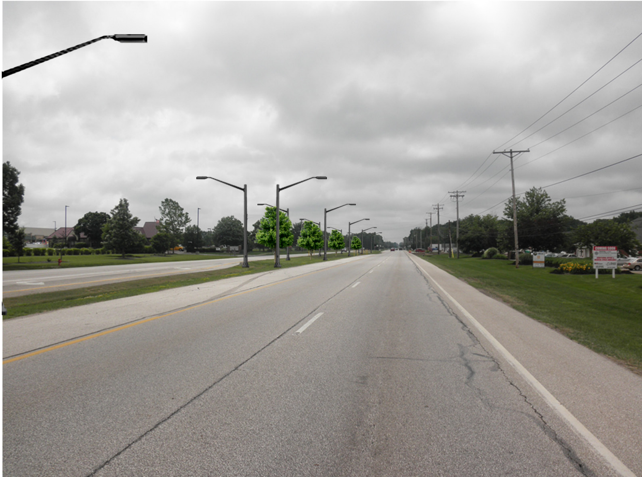
View from Corporate Drive Looking South - Day Darrow Road / SR91 Street Lighting Project Hudson, Ohio
