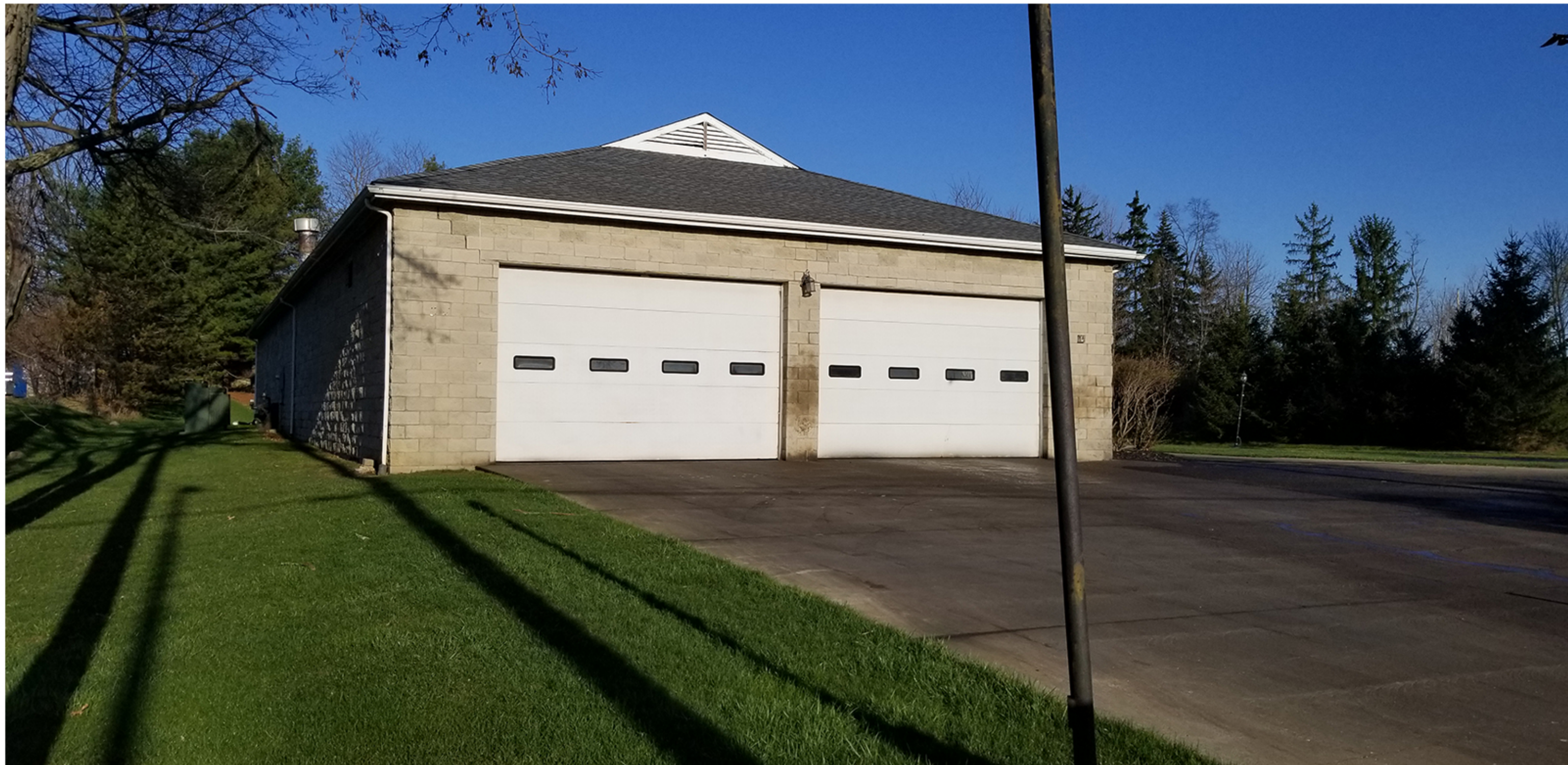
PHOTO VIEW 1 EXISTING ELEVATION (WEST / NORTH)
