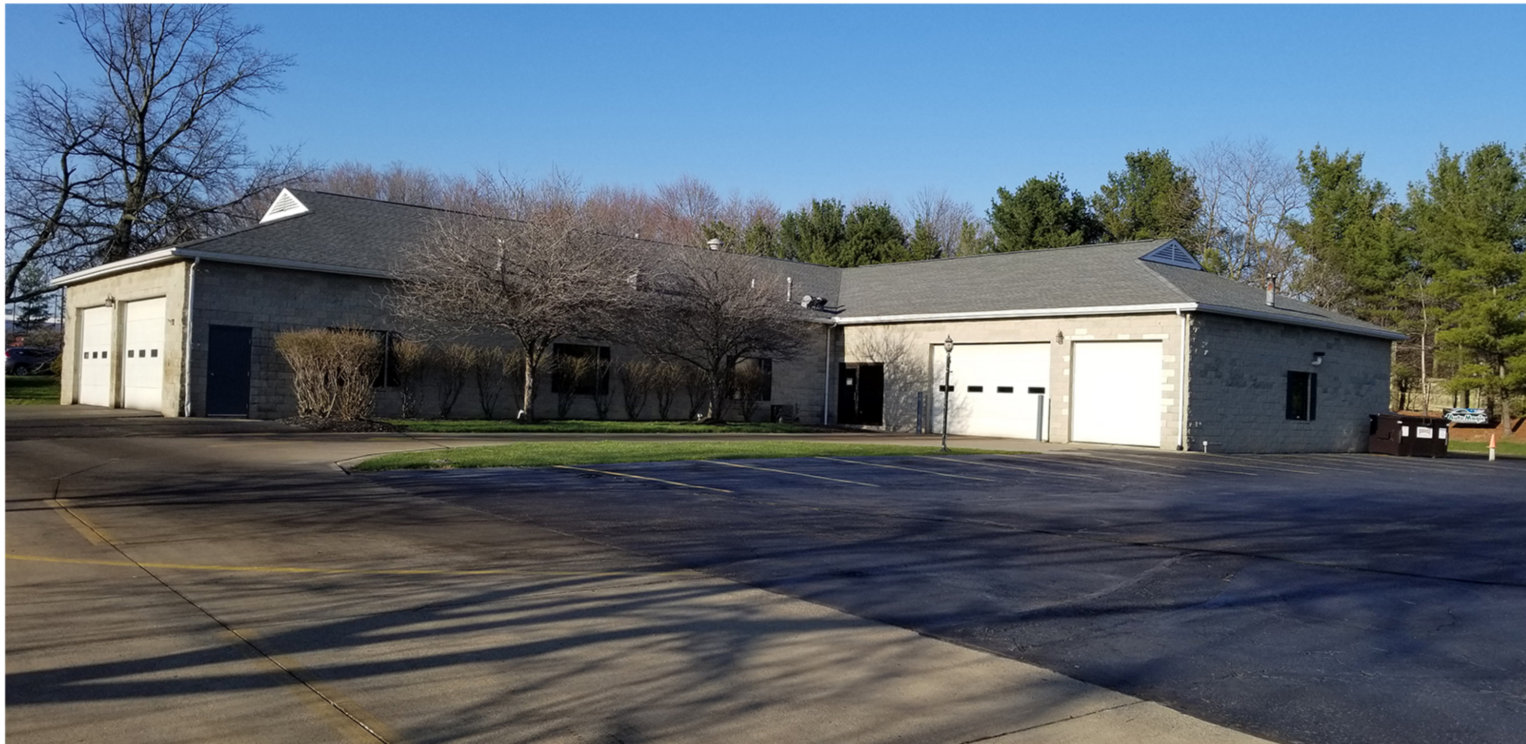
PHOTO VIEW 3 EXISTING ELEVATION (SOUTH / WEST)
