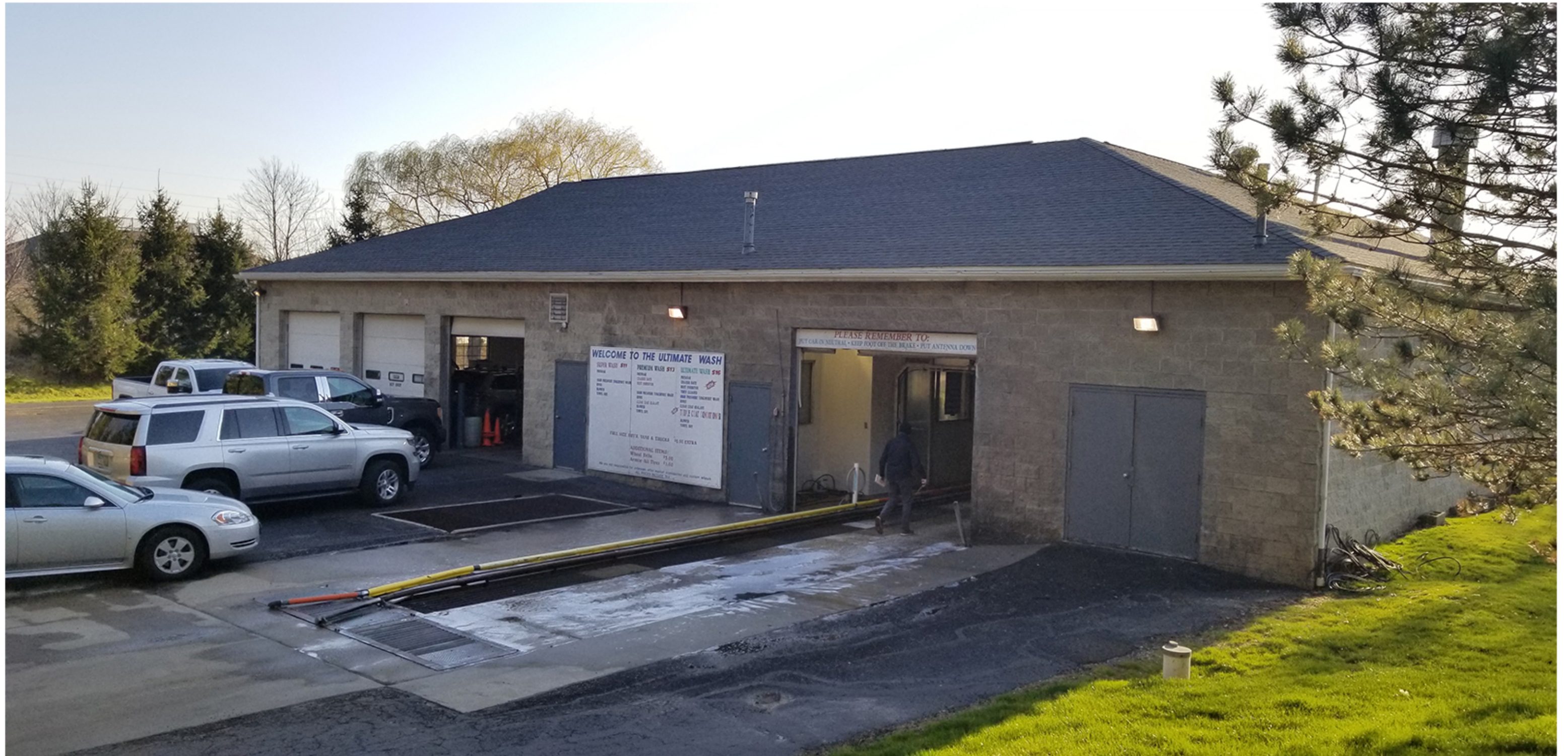
PHOTO VIEW 2 EXISTING ELEVATION (EAST)
