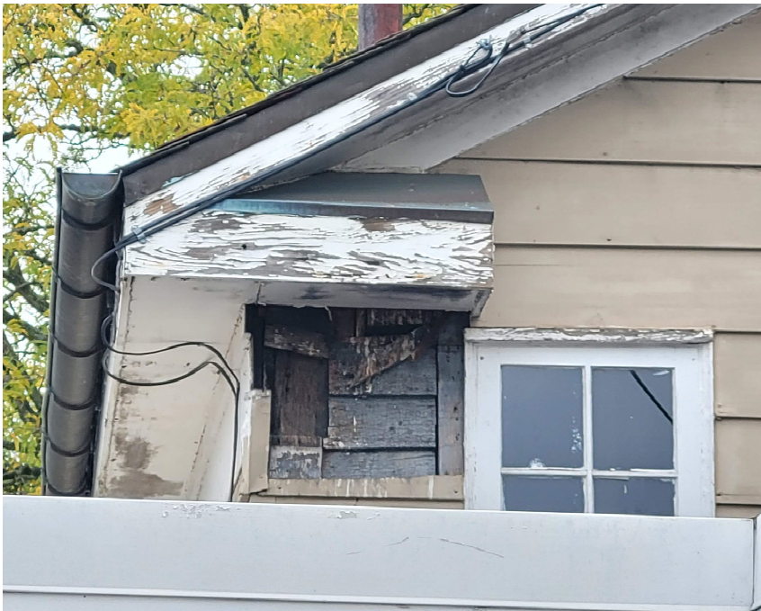
Image 9: Rear (east) elevation. Detail showing siding under existing siding. Outer layer of front elevation siding should be removed to see if another layer of wood siding exists. If so, this should be evaluated per historic photos to determine if this is the historic lap exposure width.
