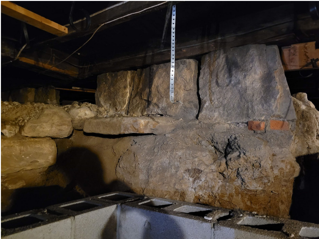
Image 13: Image taken in basement showing sandstone foundation at the north wall of the two-story portion.
