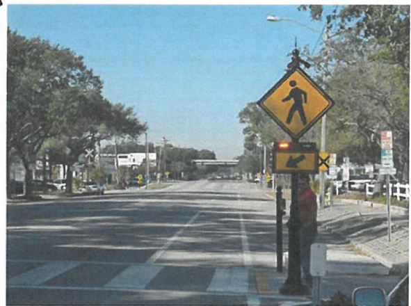
PEDESTAL MOUNTED SIGN WITH BEACONS
