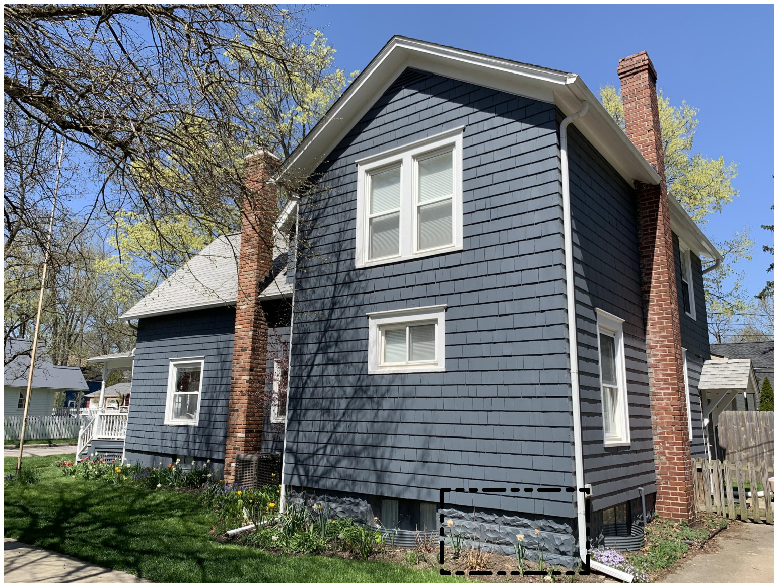
ALL NEW EXPOSED CMU FOUNDATION WALLS TO MATCH EXISTING "SPLIT FACE" BLOCK, PAINTED TO MATCH.
