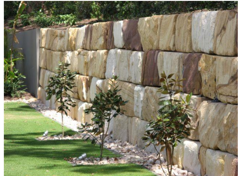
Sandstone Retaining Wall
