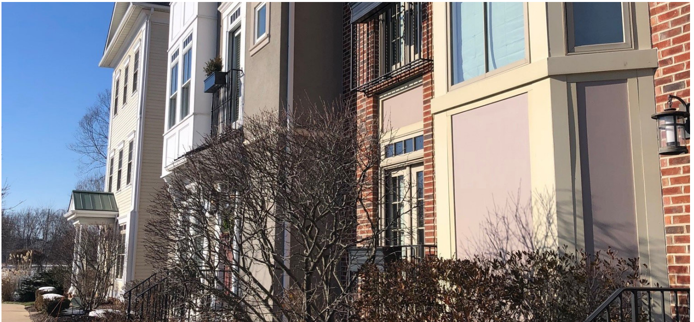
Image 3-1: Existing residential housing located in Downtown Hudson
