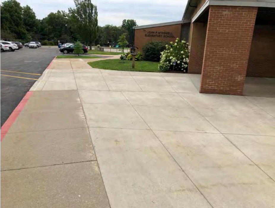
Main building entrance area
