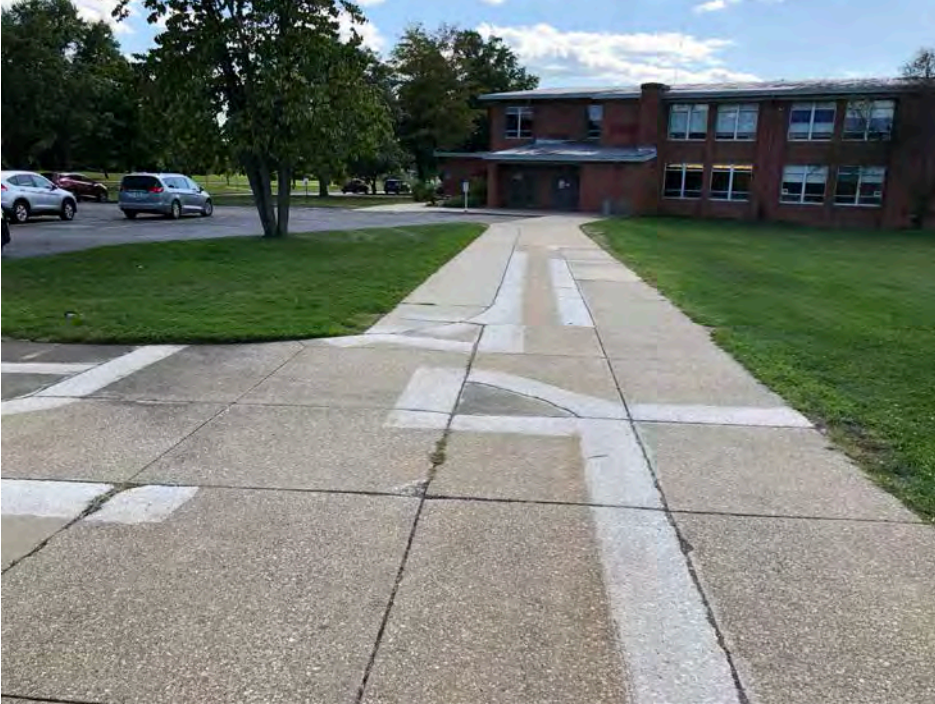
Sidewalk from McDowell to East Woods – will be removed/reconfigured
