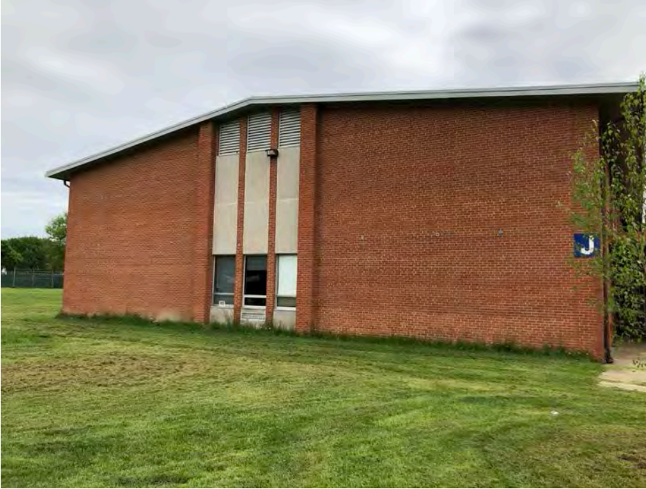
North end of 2-story wing – addition to go to the left
