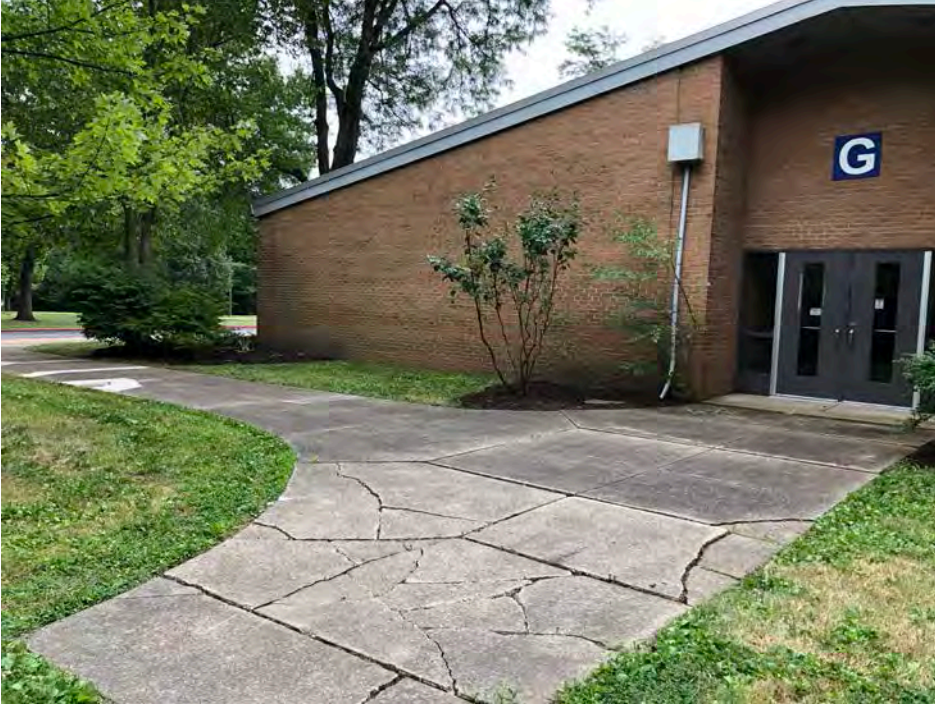
Area north of the north academic wing – sidewalk to be replaced, vegetation to remain as current
