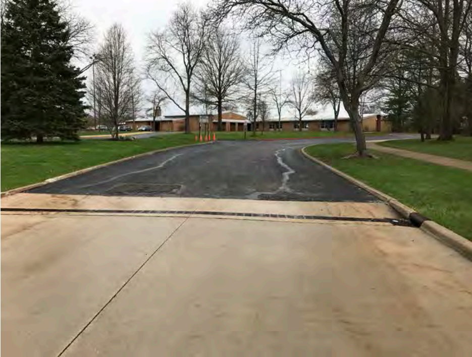
Main entrance drive from N. Hayden Pkwy. This will remain one-way in for parent arrival/dismissal
