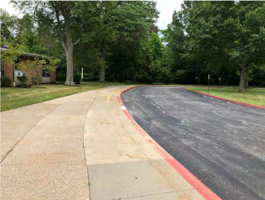
Current parent arrival/dismissal zone for both East Woods and McDowell – will now be just for McDowell. Visitor parking spaces to be provided to the right.
