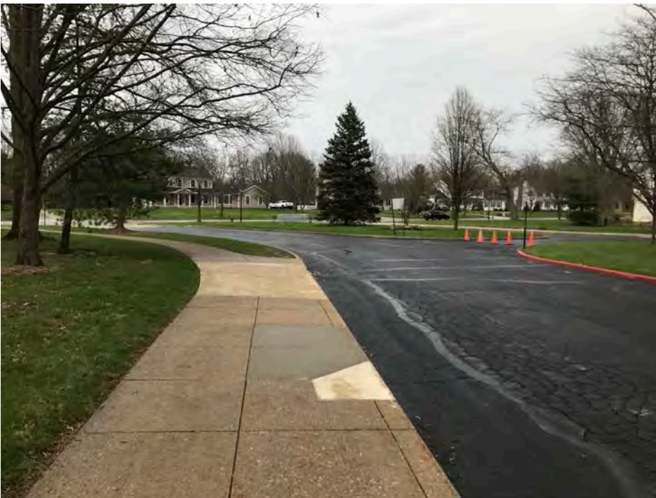
North entrance drive looking east towards N. Hayden Pkwy.
