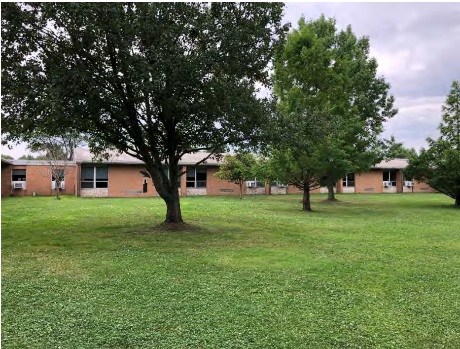
Lawn area just north of the west academic wing – to remain as current
