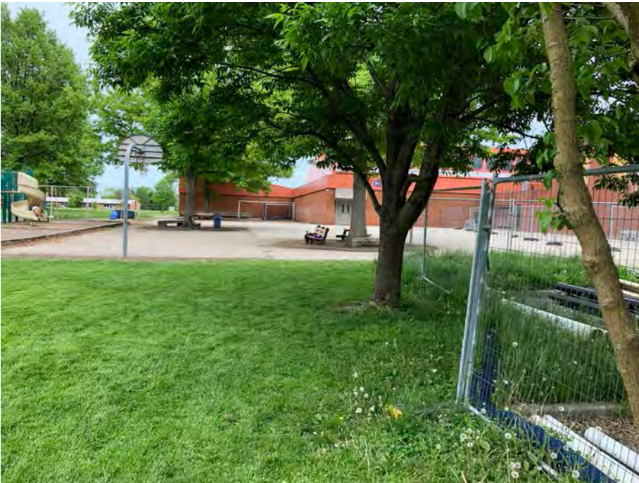
Hard surface play area. Natatorium construction ongoing to the right
