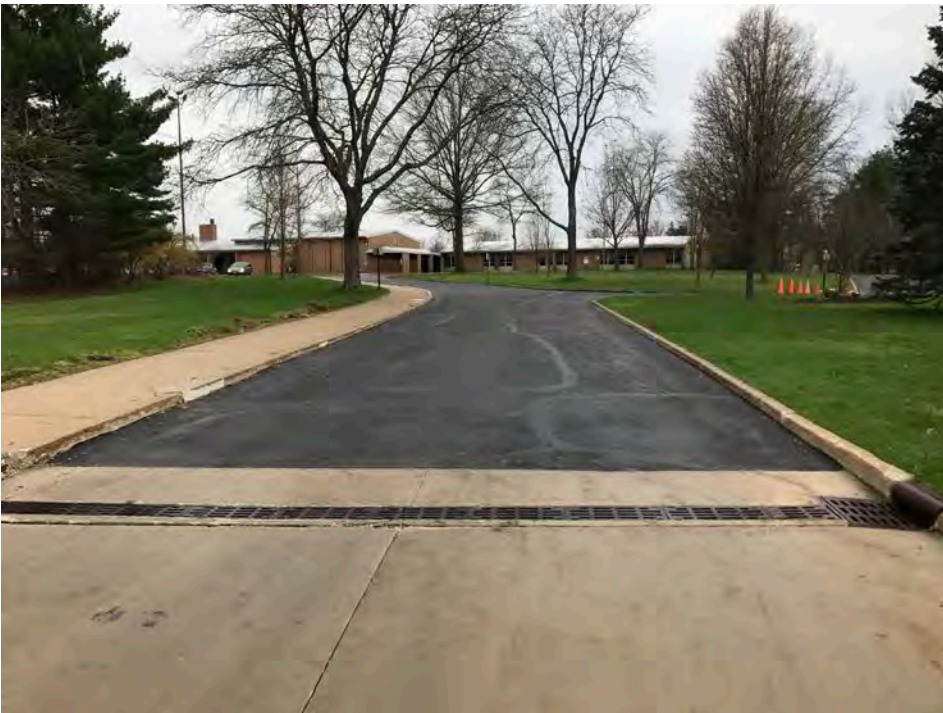
South drive currently one-way out. This drive will be widened for one lane in and 2 lanes out (left/right turn)
