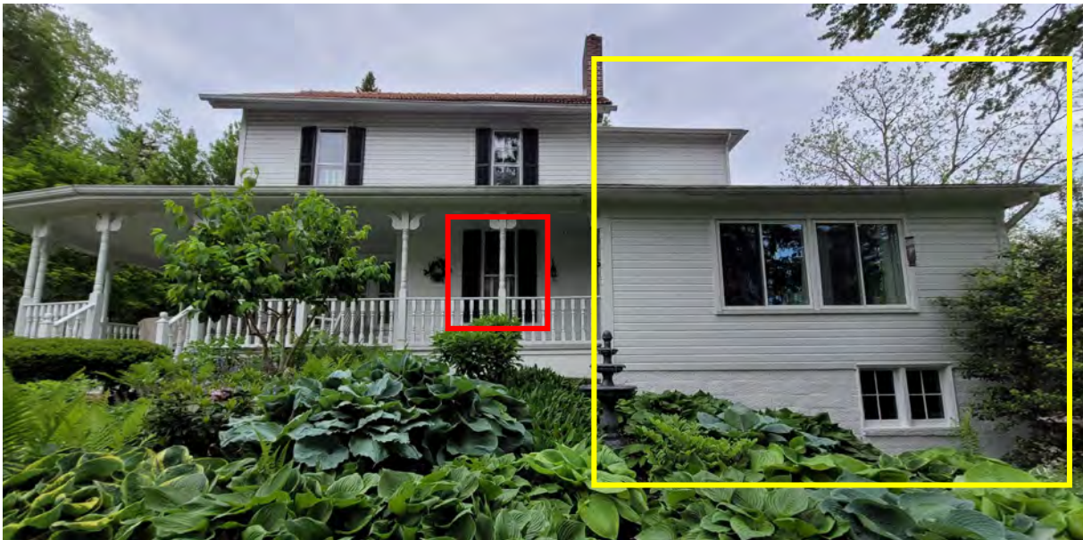
Image 4: Side, southwest, elevation. The red box indicates the window to be removed. The yellow box indicates the previous addition to be removed.
