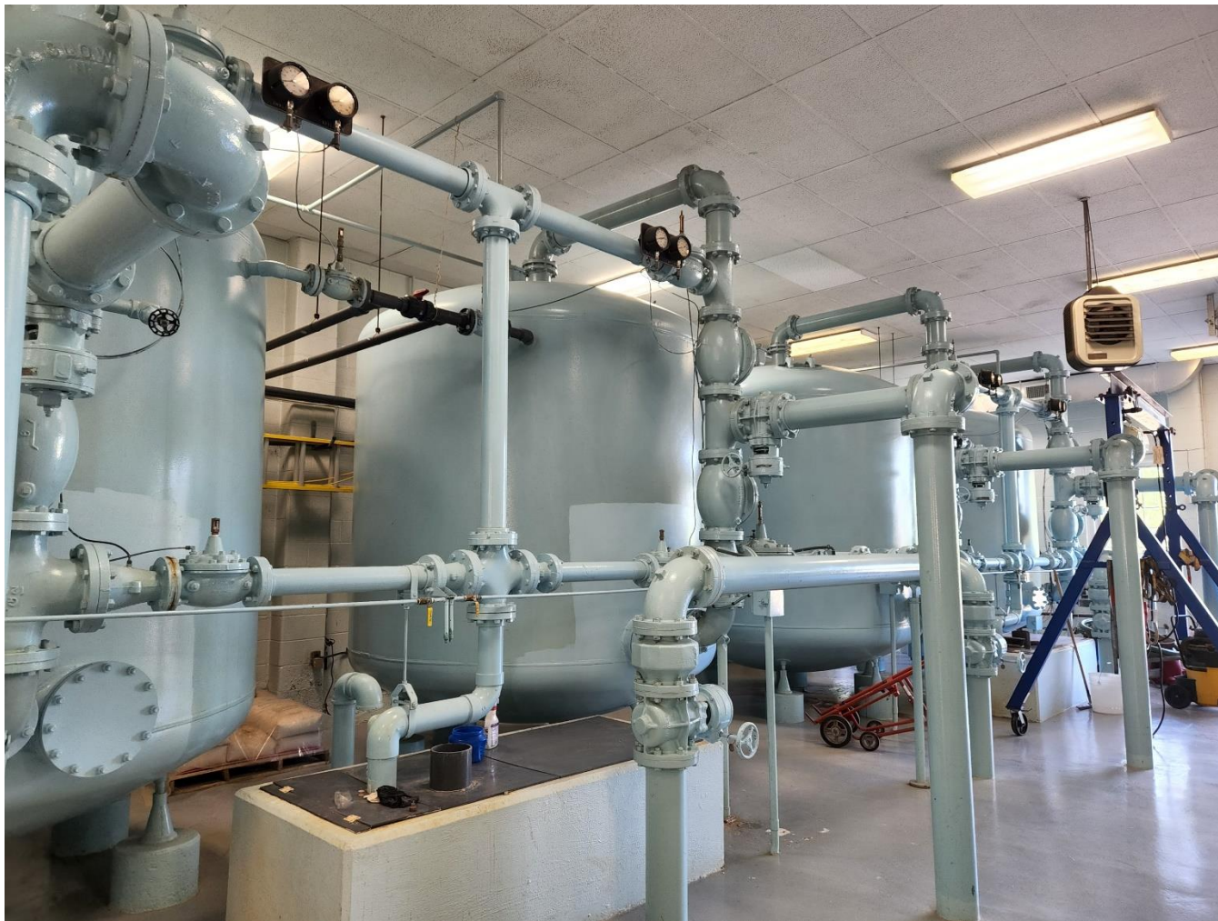
Figure 16. Photo of four ion-exchange water softeners at Hudson Water Treatment Plant
