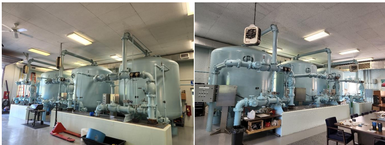
Figure 14. Photo of six filters at the Hudson Water Treatment Plant
