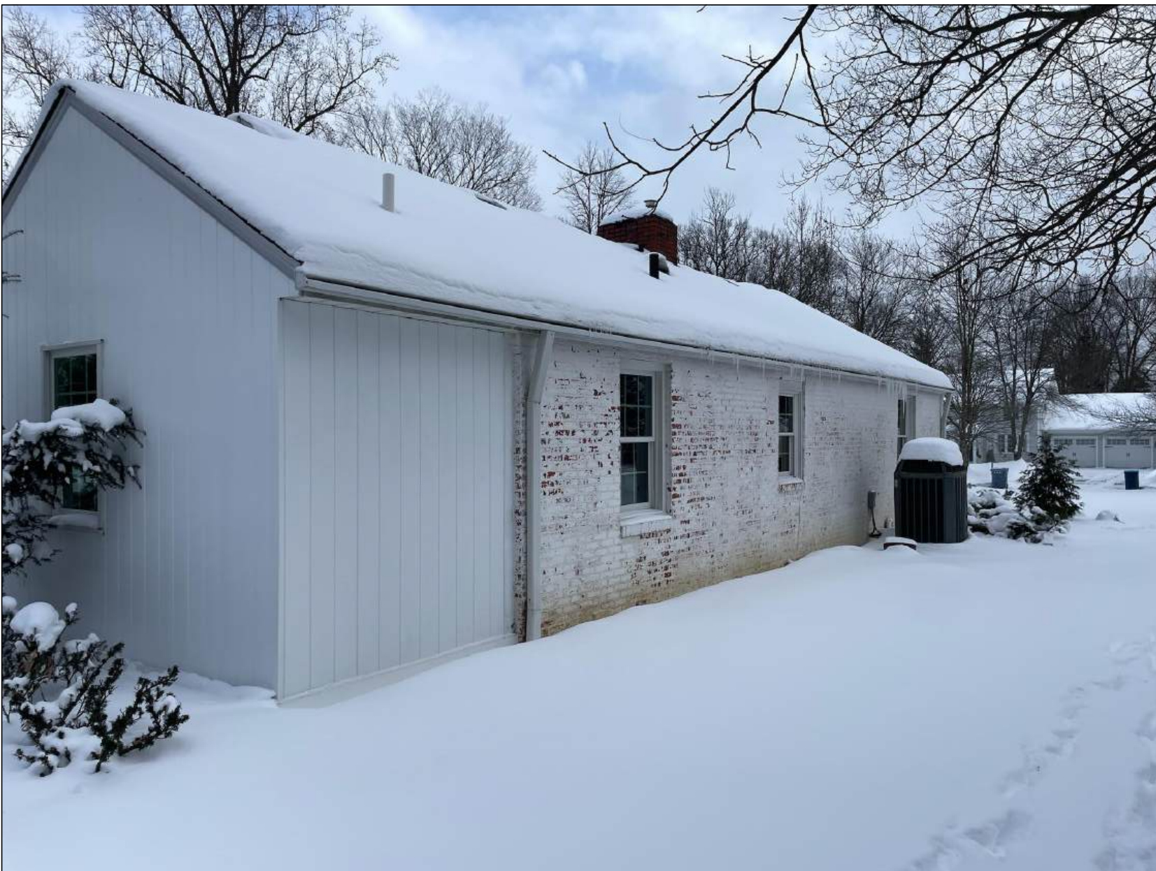
existing house - rear n.w. corner
