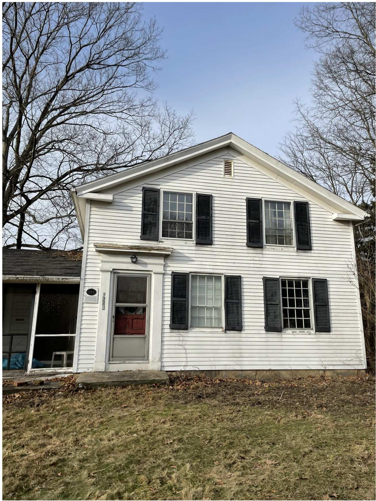
IMAGE OF THE EXISTING HOUSE FOR REFERENCE - S
