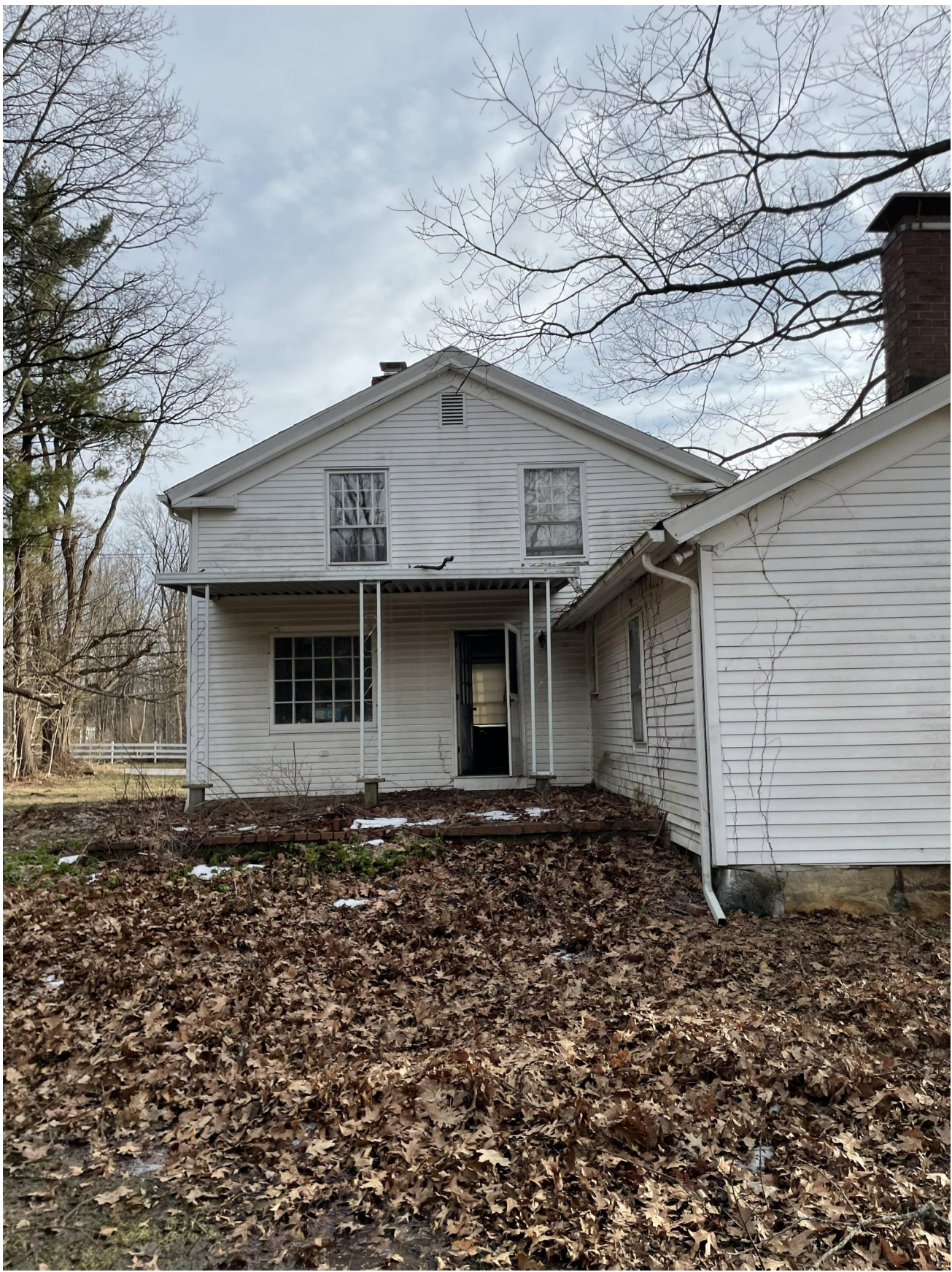
IMAGE OF THE EXISTING HOUSE FOR REFERENCE - N
