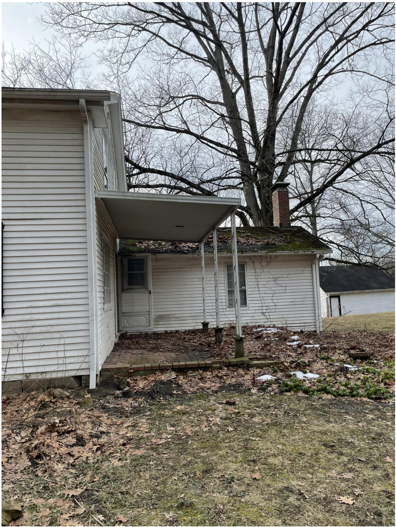
IMAGE OF THE EXISTING HOUSE FOR REFERENCE - E
