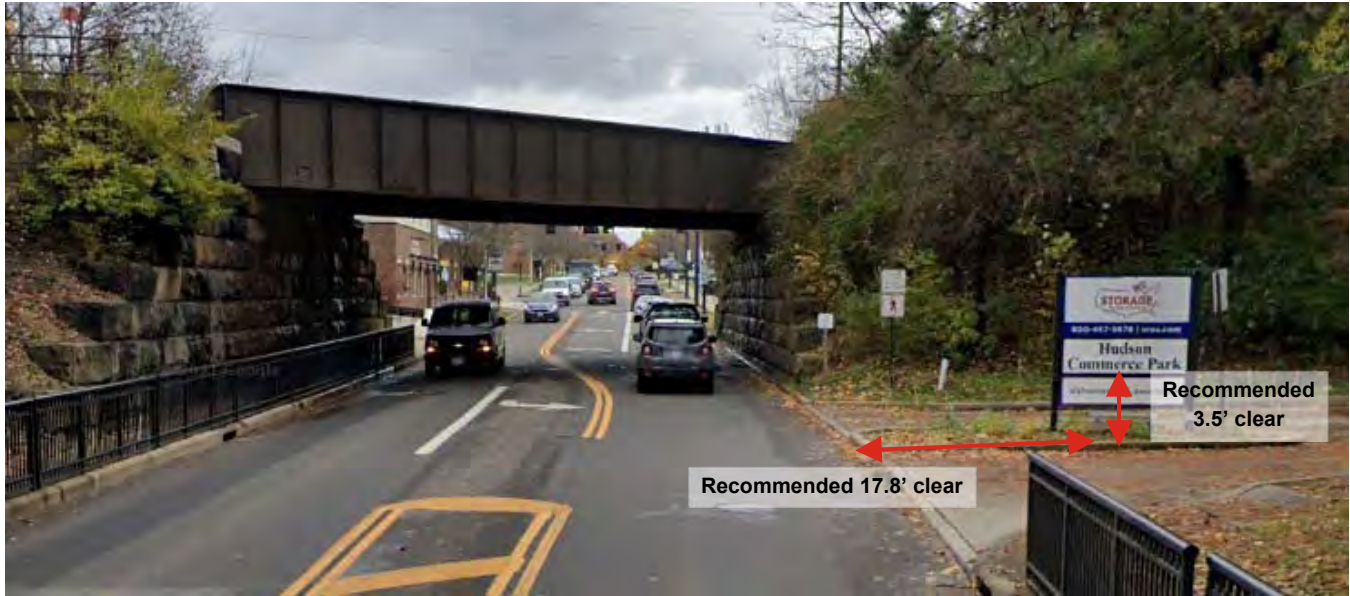
Figure 4: Sign blocking sight distance
