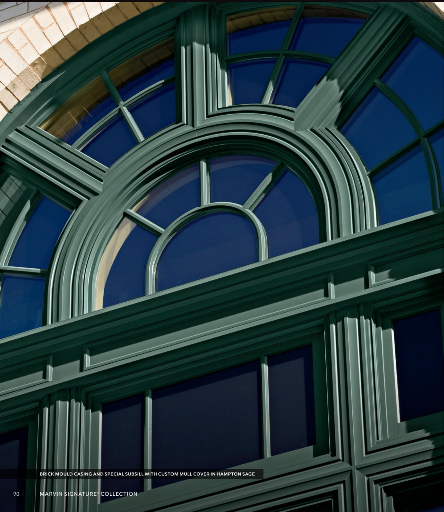
BRICK MOULD CASING AND SPECIAL SUBSILL WITH CUSTOM MULL COVER IN HAMPTON SAGE
