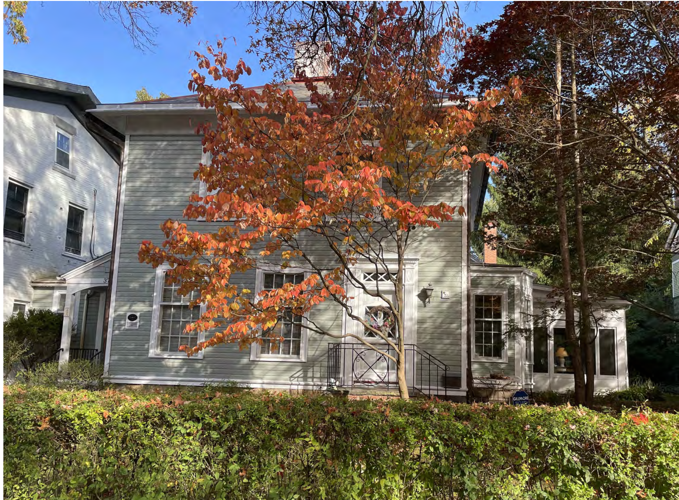
WEST ELEVATION - SHOWING SUN PORCH
