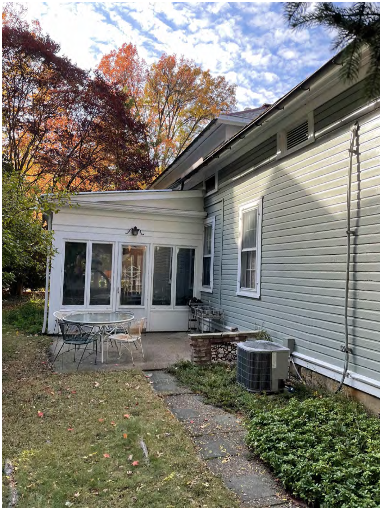
SOUTH ELEVATION - FROM BACK YARD
