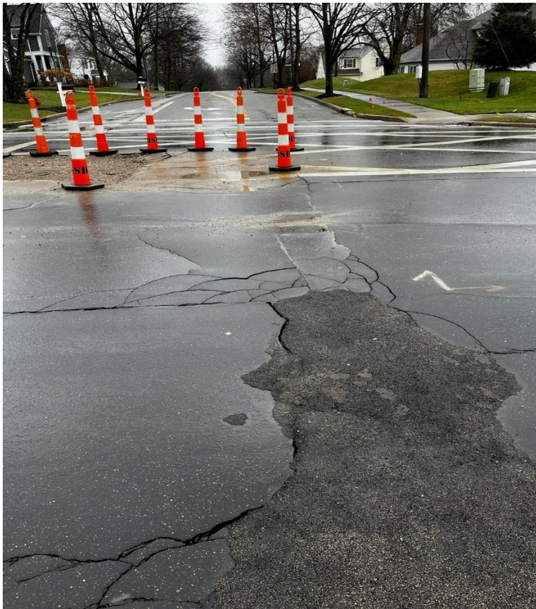
303 looking North Down Lennox
