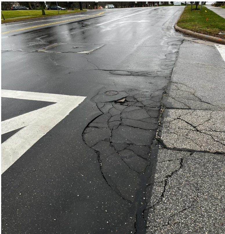
303 at Lennox looking West
