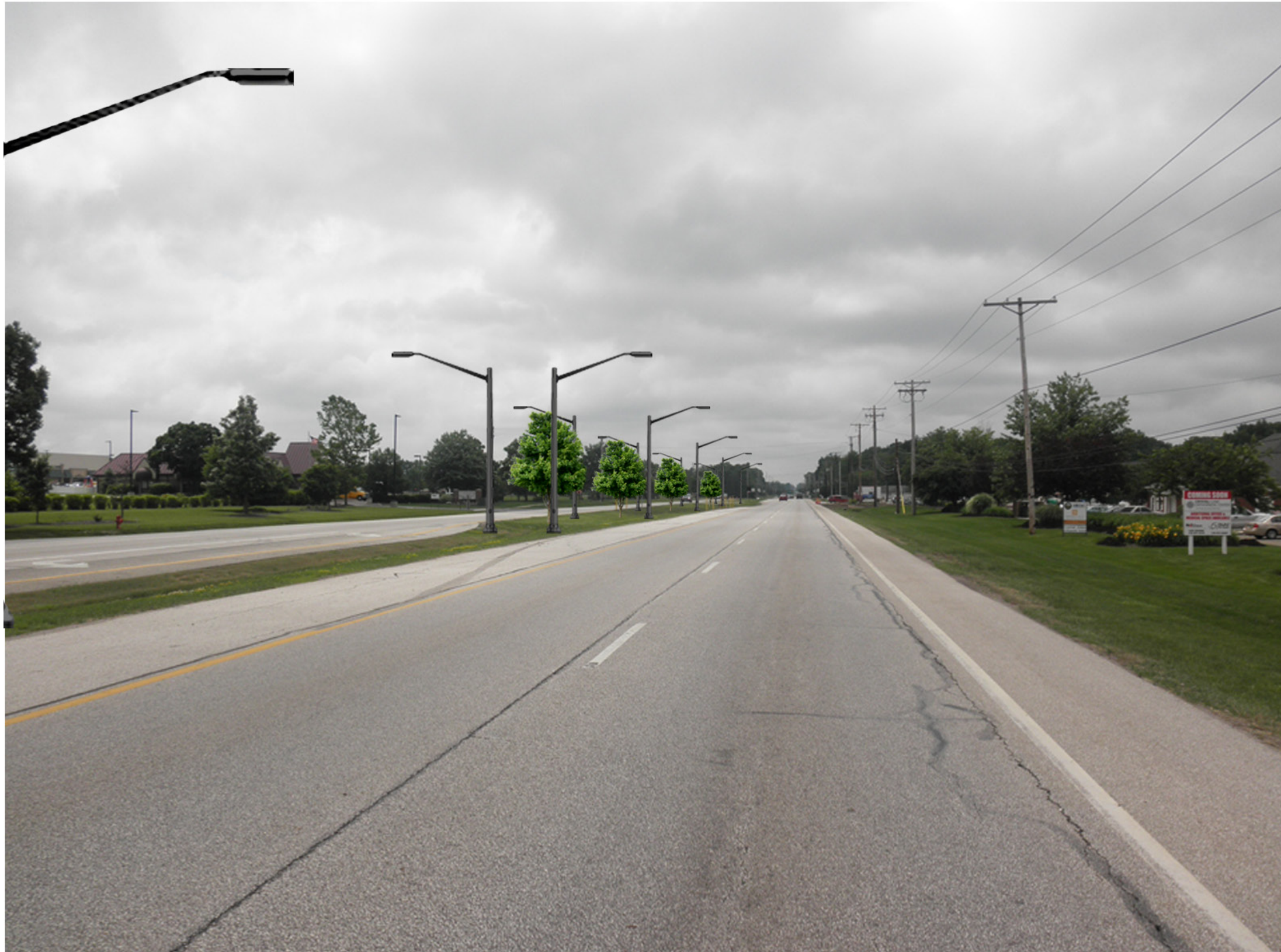
View from Corporate Drive Looking South - Day Darrow Road / SR91 Street Lighting Project Hudson, Ohio
