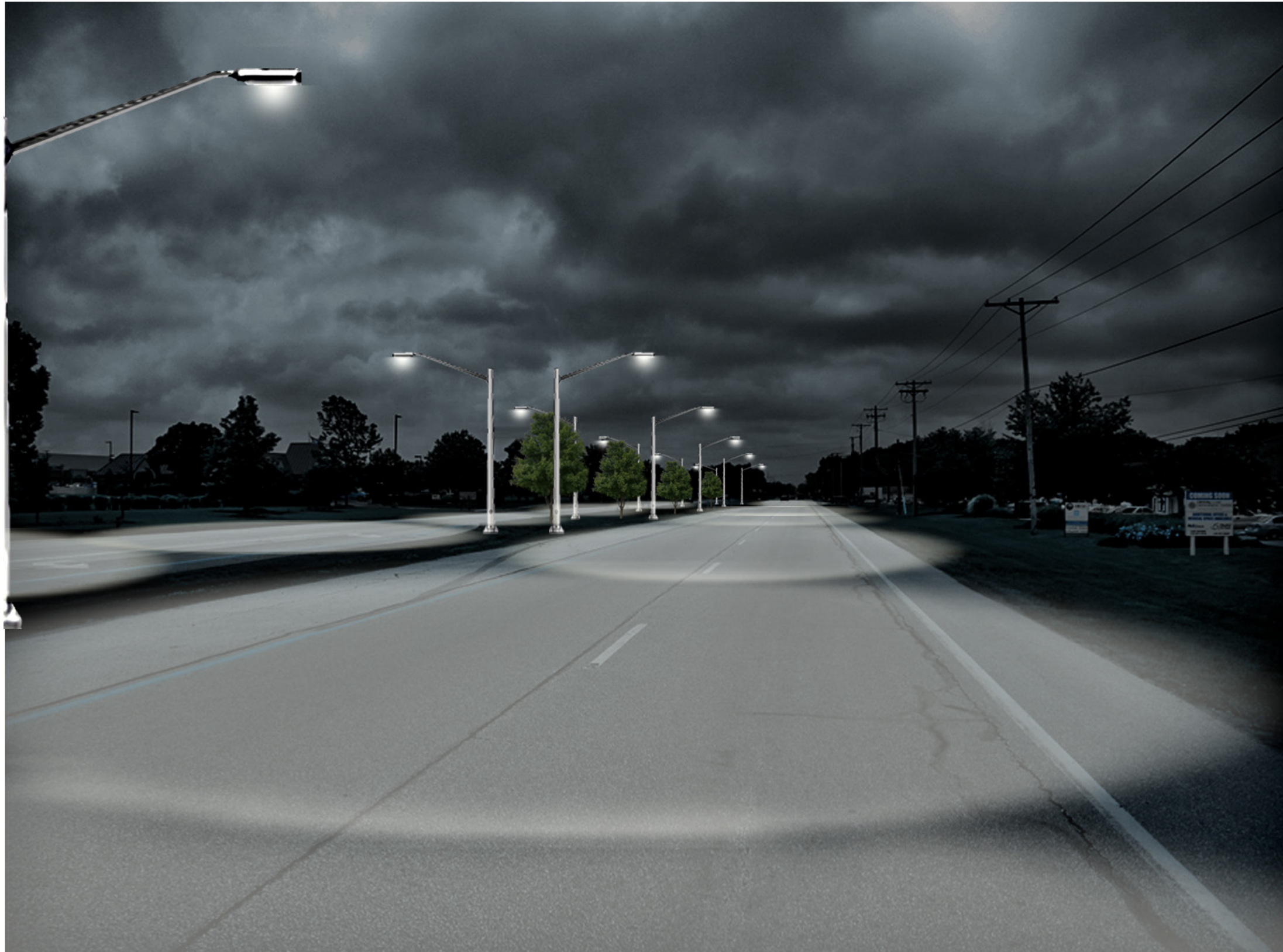
View from Corporate Drive Looking South - Night Darrow Road / SR91 Street Lighting Project Hudson, Ohio
