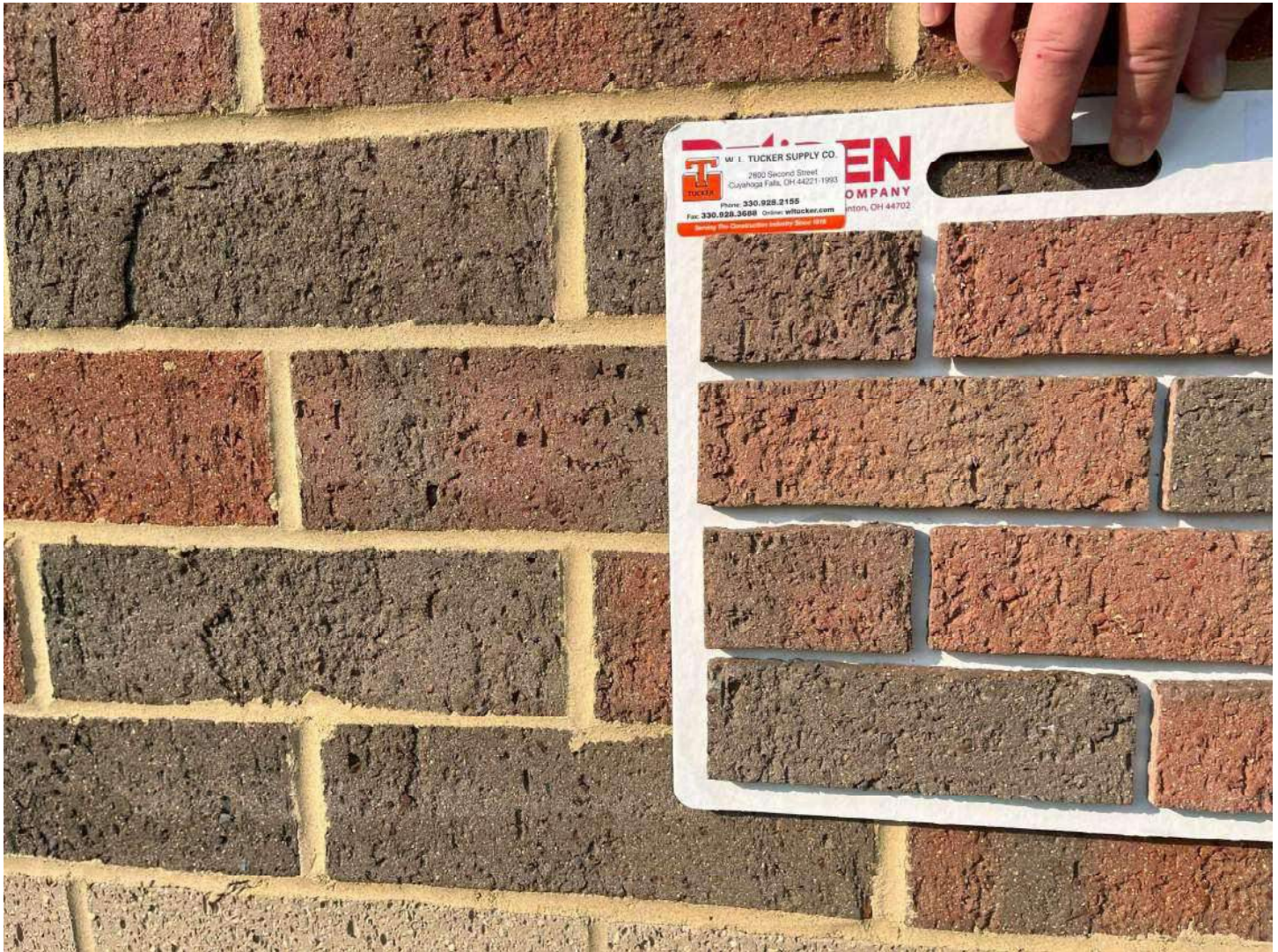
Brick Type 1 held up against existing field brick (Belden Tudor Blend Dart-TeX)
