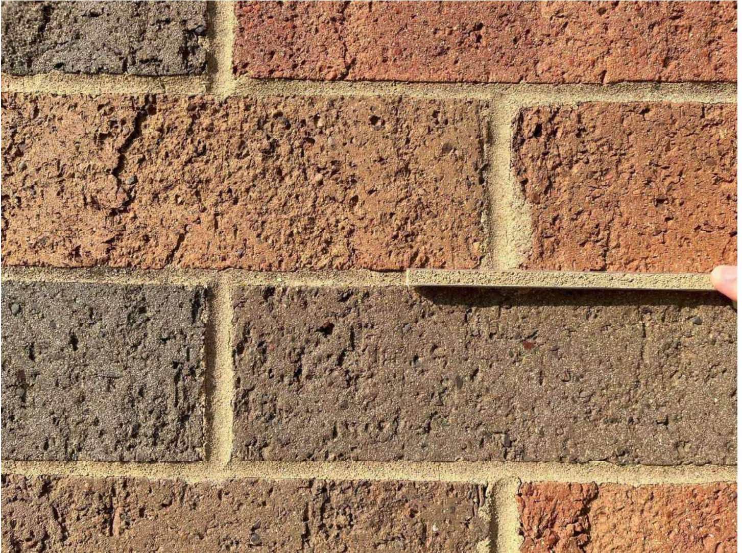
Mortar selection for field brick Type 1 (Fairborn Cement Company – 55C Keystone)
