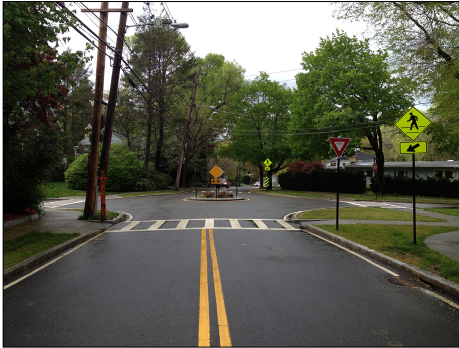
Figure 5: Example of mini roundabout within intersection
