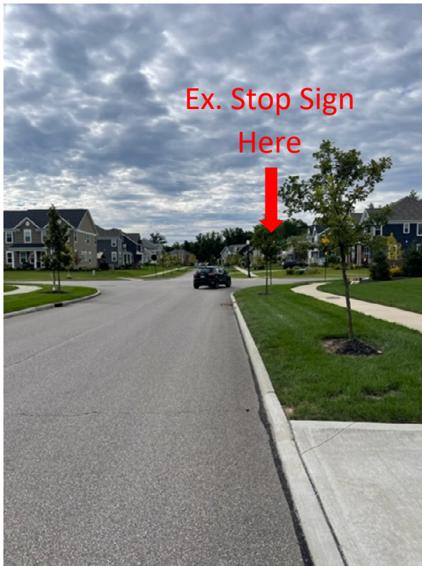
Figure 1: Timberline Trail Looking South
