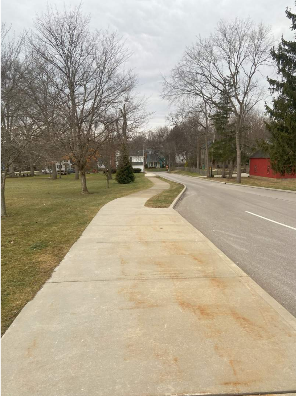
Hudson Middle School entrance drive looking west. The 34-foot wide drive and 10-foot wide pedestrian path installed during the middle school construction merges to the original 20-foot wide drive and 5'-6" wide sidewalk north of the Saywell House.
