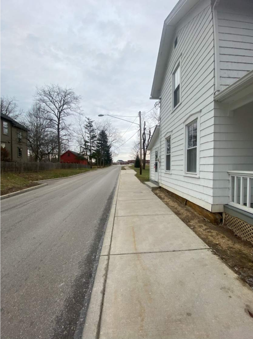
Entrance drive looking east between 91 N. Oviatt Street and the Saywell House (77 N. Oviatt St.). The drive is currently 20-feet wide with a 5'-6" wide sidewalk.
