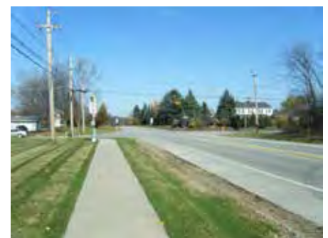
Sidewalk along Stow Road in front of Ellsworth Hill Elementary
