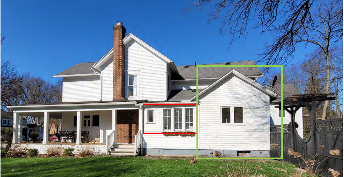
Image 6: Side (east) elevation. The red box indicates the historic pre-1950 windows to be removed. The green box indicates the pre-1950 historic addition side gable to be removed.
