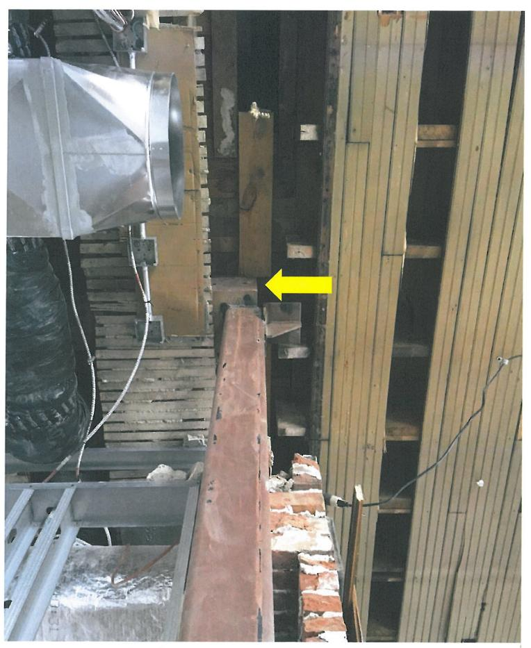
17. New Steel Tube Supports 12"x12" Wood Timber Beam
