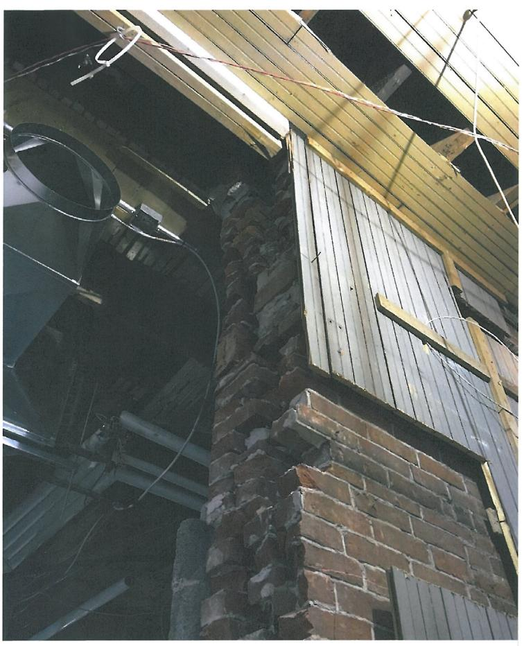
9. Existing East Brick Wall at Fire Museum Entrance (North) View looking west. Brick wall and wood floor joists above are supported by thin 2"x4" wood framing
