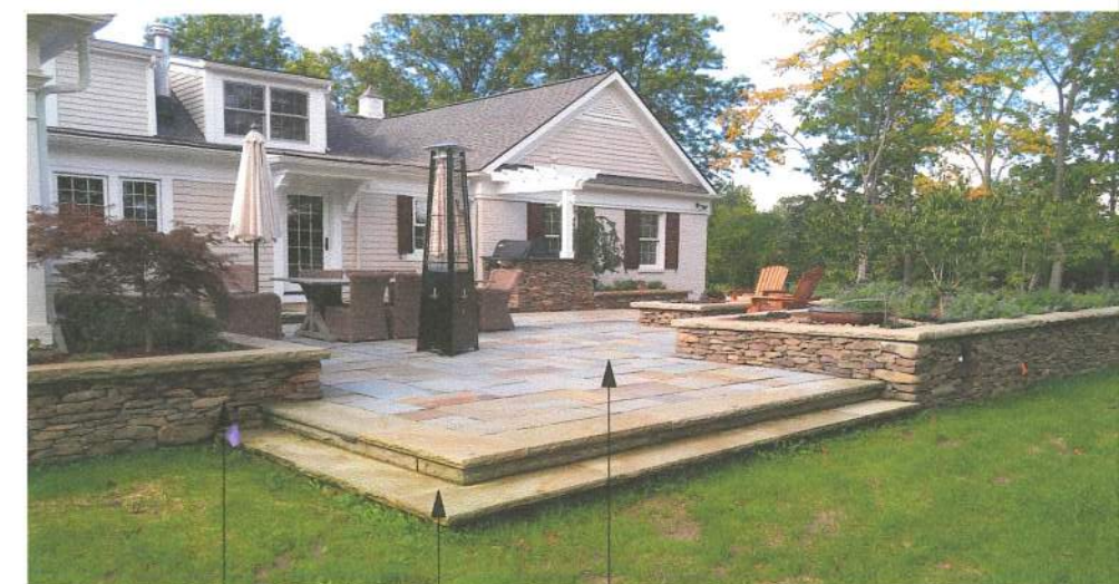
Dry Laid Blue Stone Patio Materials Sandstone Steps w/ Field Stone Riser Materials Field Stone Retaining Wall w/ Sandstone Cap Materials
