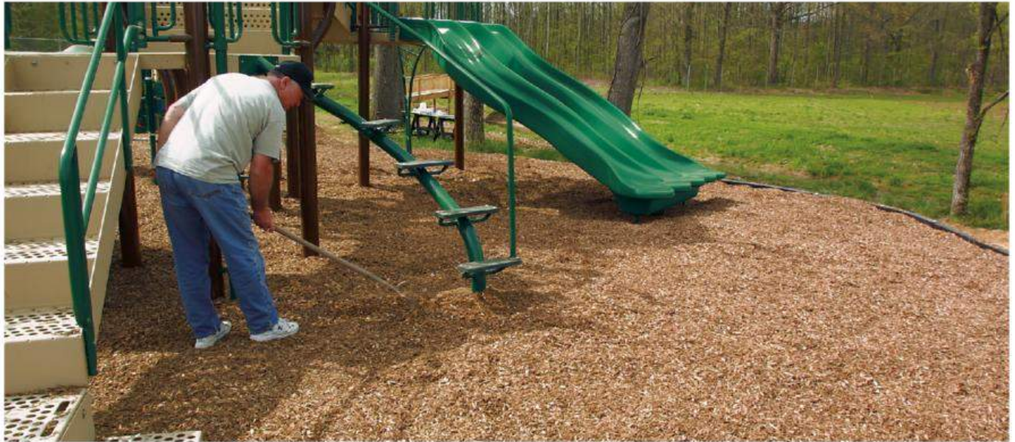
Raking loose-fill engineered wood fiber material
