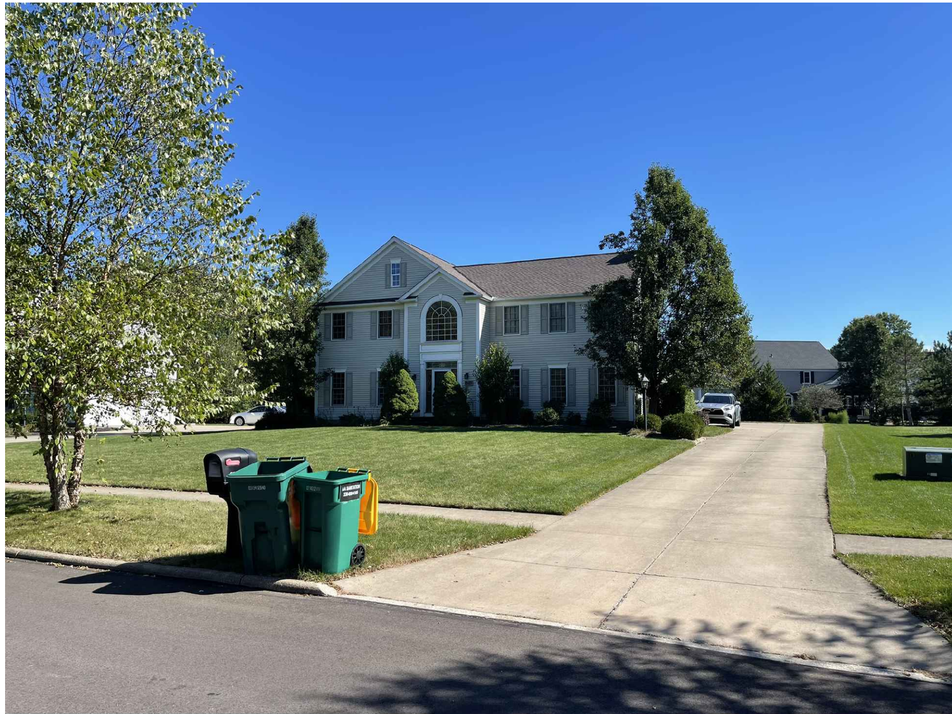
8 - NEIGHBORING PROPERTY TO THE SOUTH (5731 NOTTINGHAM GATE BLVD.)
