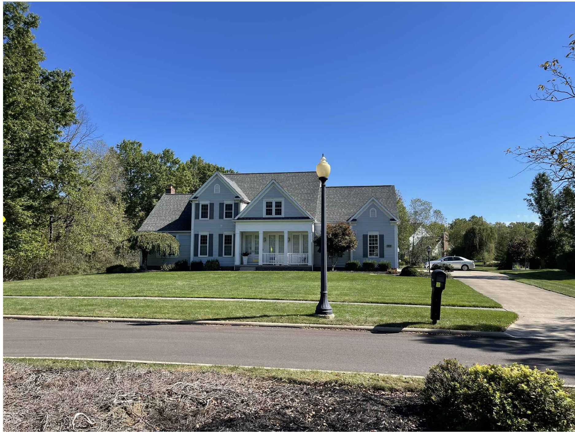
7 - NEIGHBORING PROPERTY TO THE SOUTH (5743 NOTTINGHAM GATE BLVD.)
