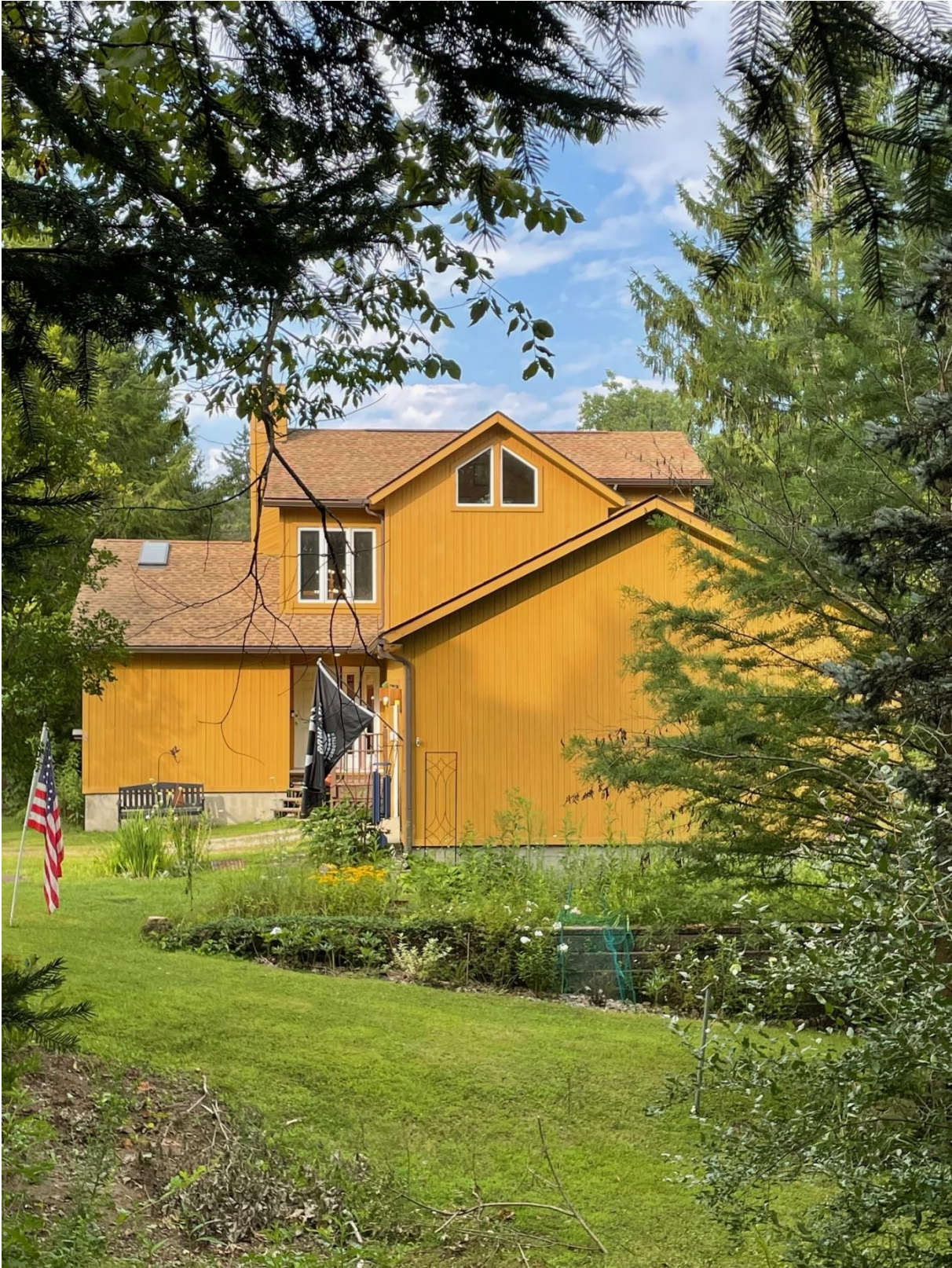
East Elevation View
