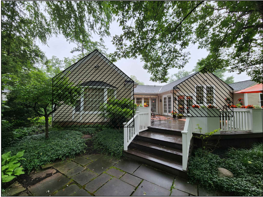
AREA OF SOUTH ELEVATION WHERE NEW ADDITION IS PROPOSED
