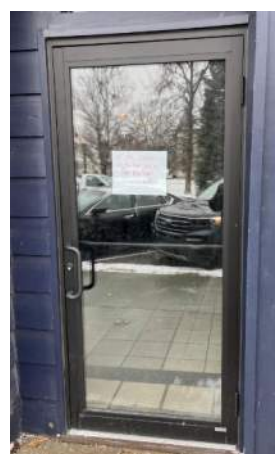
Front door after replacement
