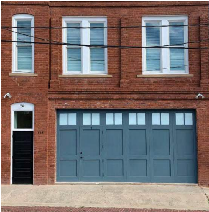
Figure 20. Cement board was used to replace a non-historic infill and mimics the configuration of a typical vehicular door of the period. Photos: Historic Augusta.
