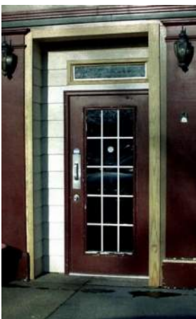
Front door before replacement
