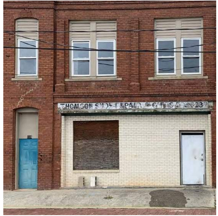
Figure 20. Cement board was used to replace a non-historic infill and mimics the configuration of a typical vehicular door of the period. Photos: Historic Augusta.
