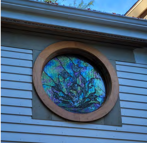
Image 1: Circular art glass window to be moved. Note the rough framing vertical boards around the window.
