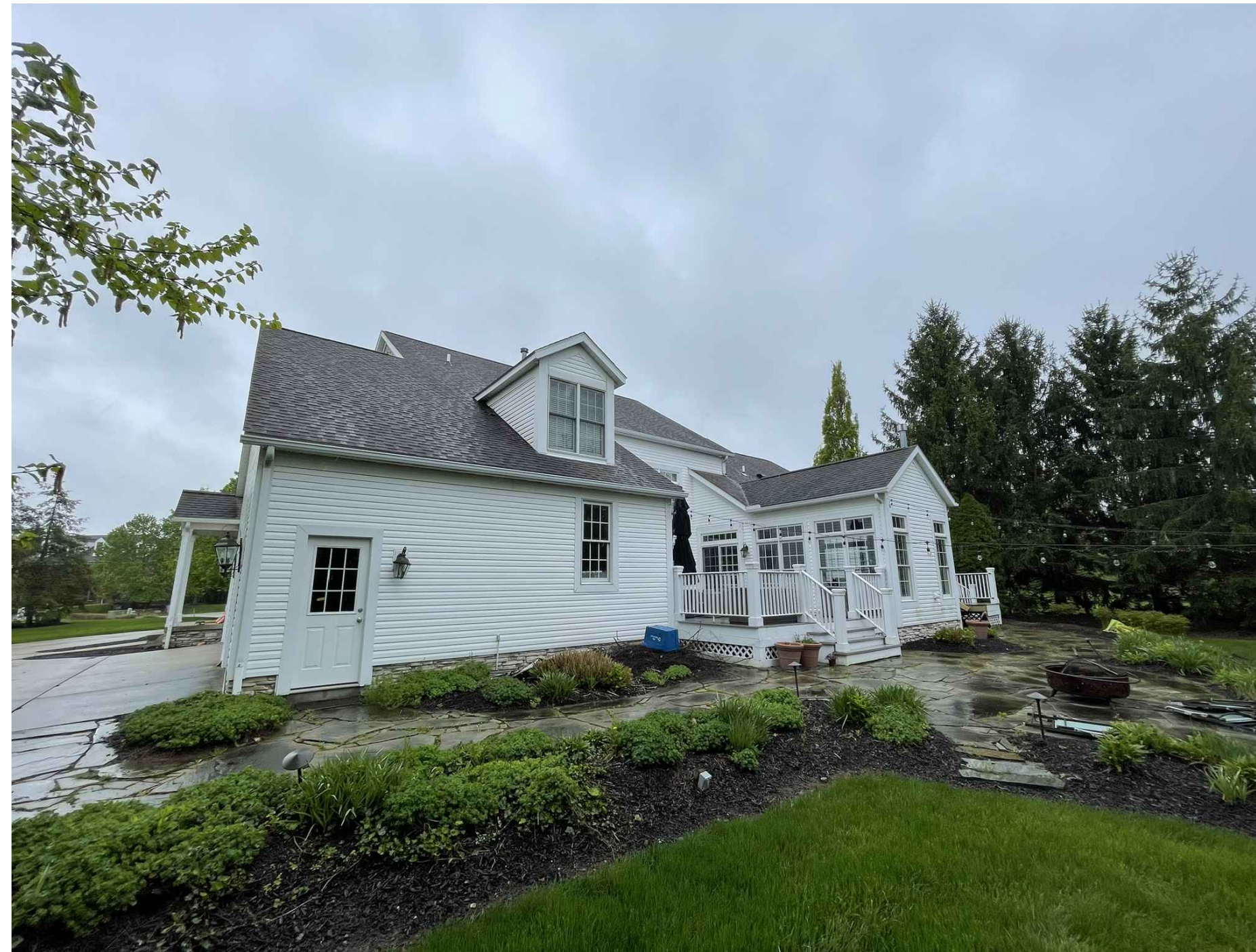
5 - REAR OF HOUSE (WEST)
