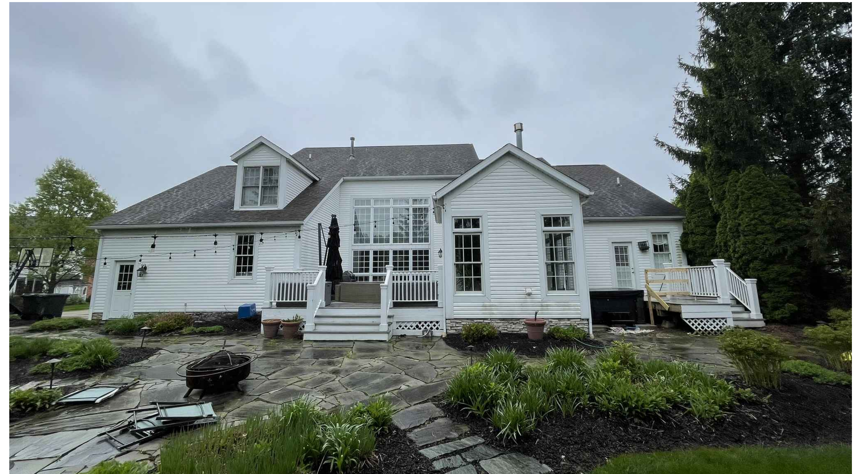
REAR OF HOUSE (WEST), EXISTING
