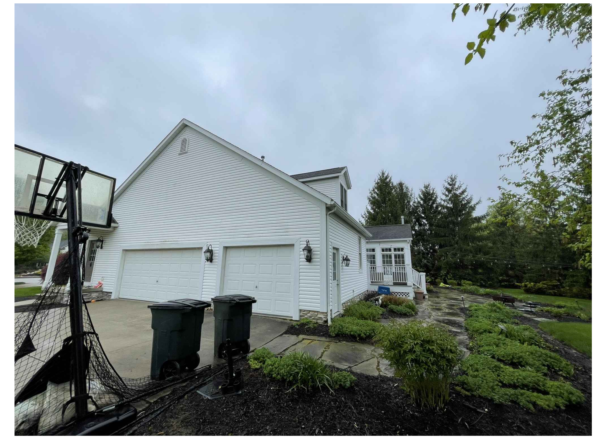
3 - SIDE OF HOUSE (NORTH)
