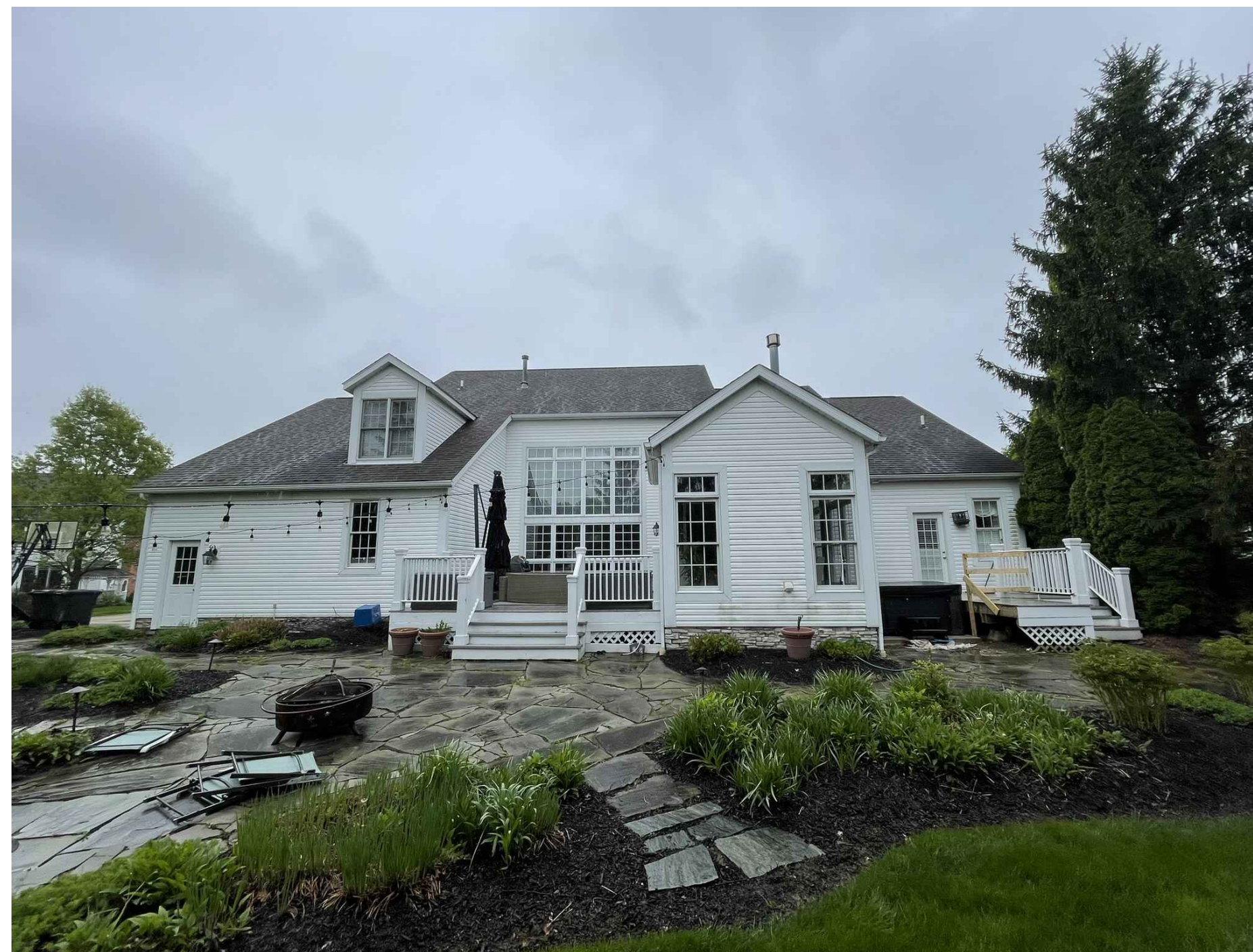
4 - REAR OF HOUSE (WEST)
