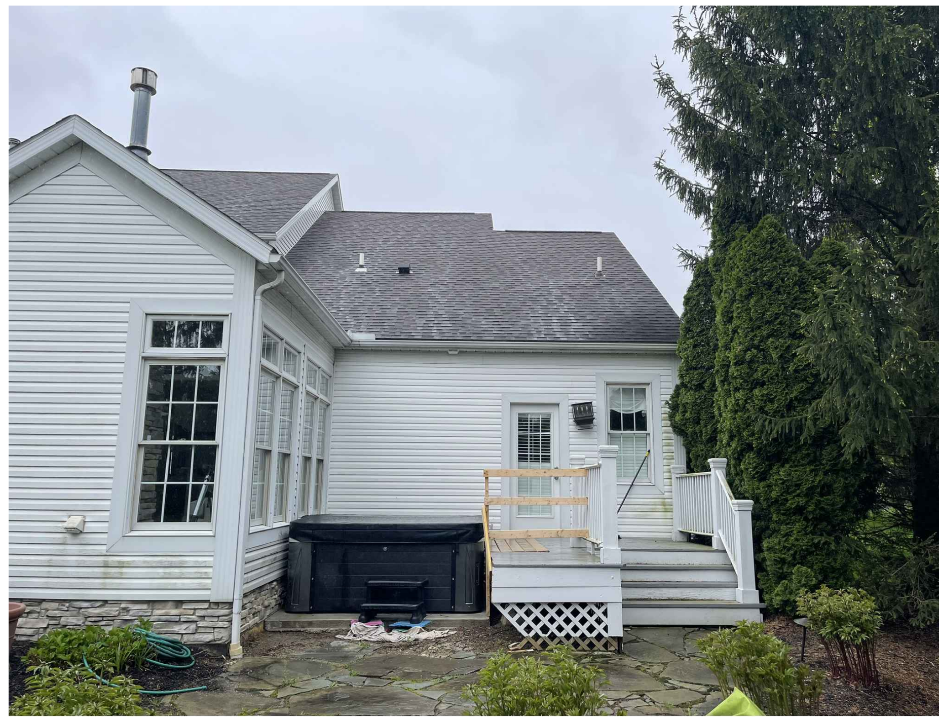
6 - REAR OF HOUSE (WEST)
