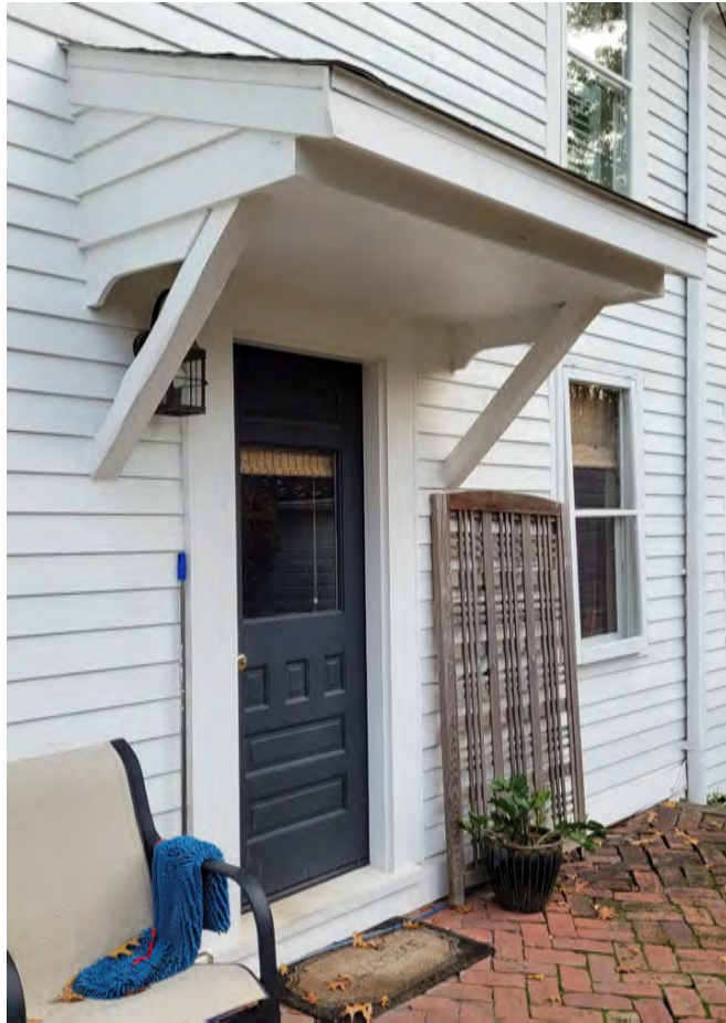
Image 4: Detail view of non-historic wood door in presumed historic location/opening with non-historic shed roof overhang.
