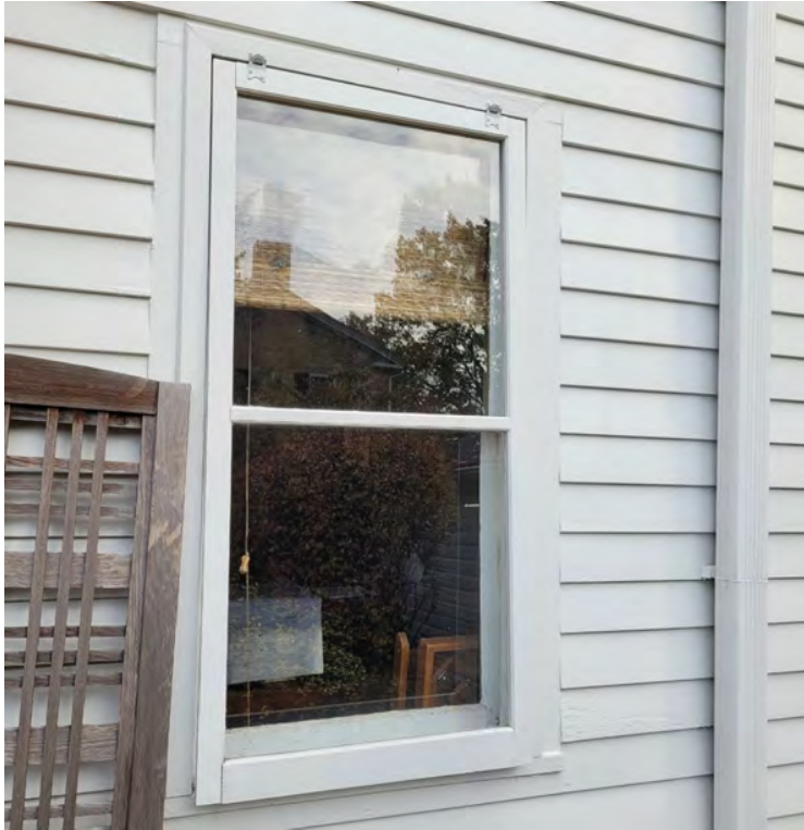
Image 2: Detail view of one of the historic first-floor wood windows with presumed historic storm window to be removed.
