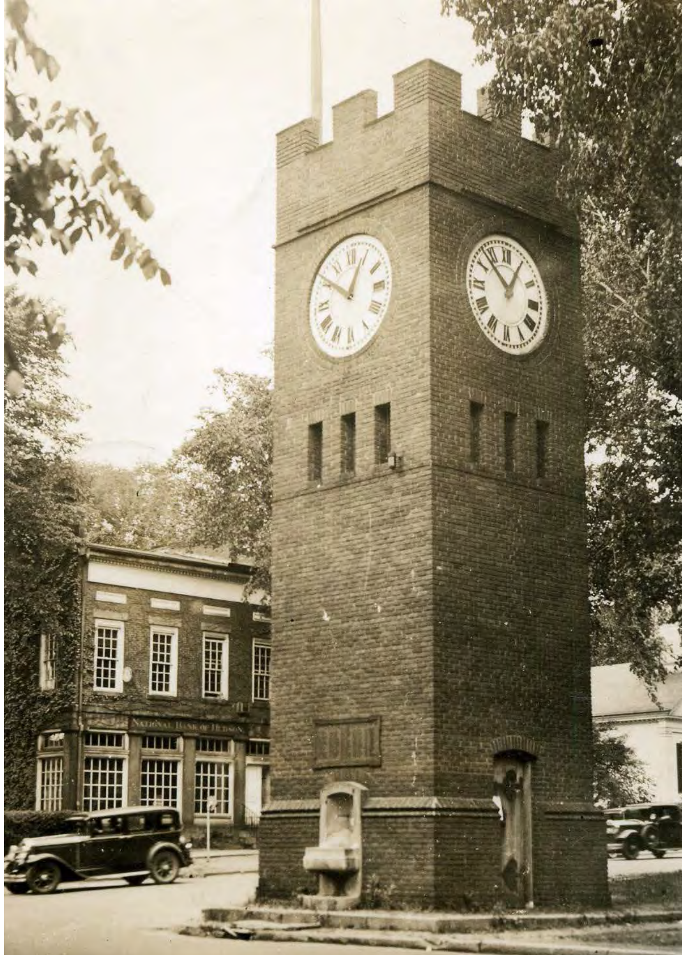
West elevation of Clock Tower with original WWI Memorial Bronze Tablet, ca.1920s
