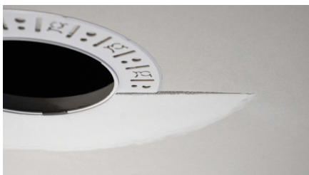
Partially finished mud ring, showing cross-section detail.
