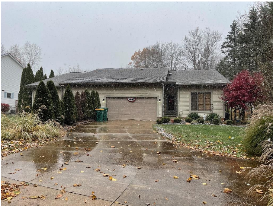
253/255 Ravenna Street – Same Side of Street
