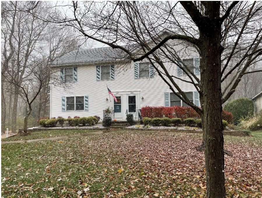
247/249 Ravenna Street – Same Side of Street
