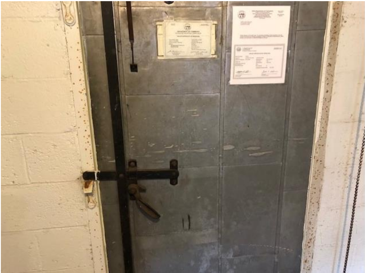
Figure 9 - possible SAFE ROOM - Boiler room
