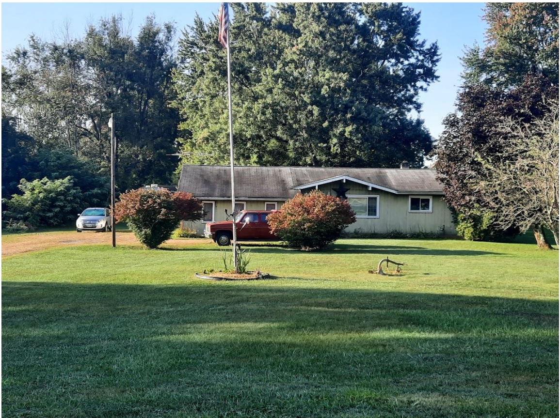
760 Barlow Road – 2 nd house east of project site.
