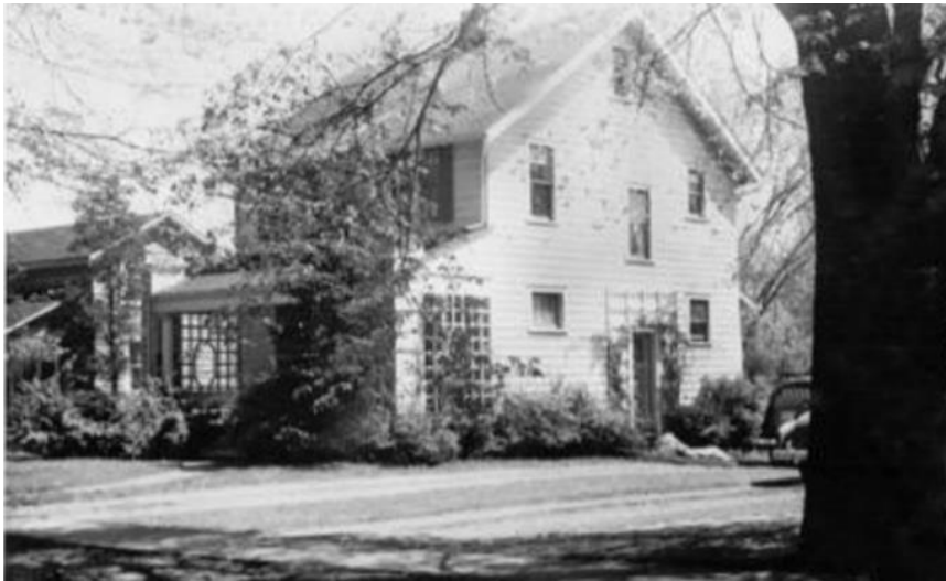
Figure 20. 152 Elm Street House, Photo 1950
