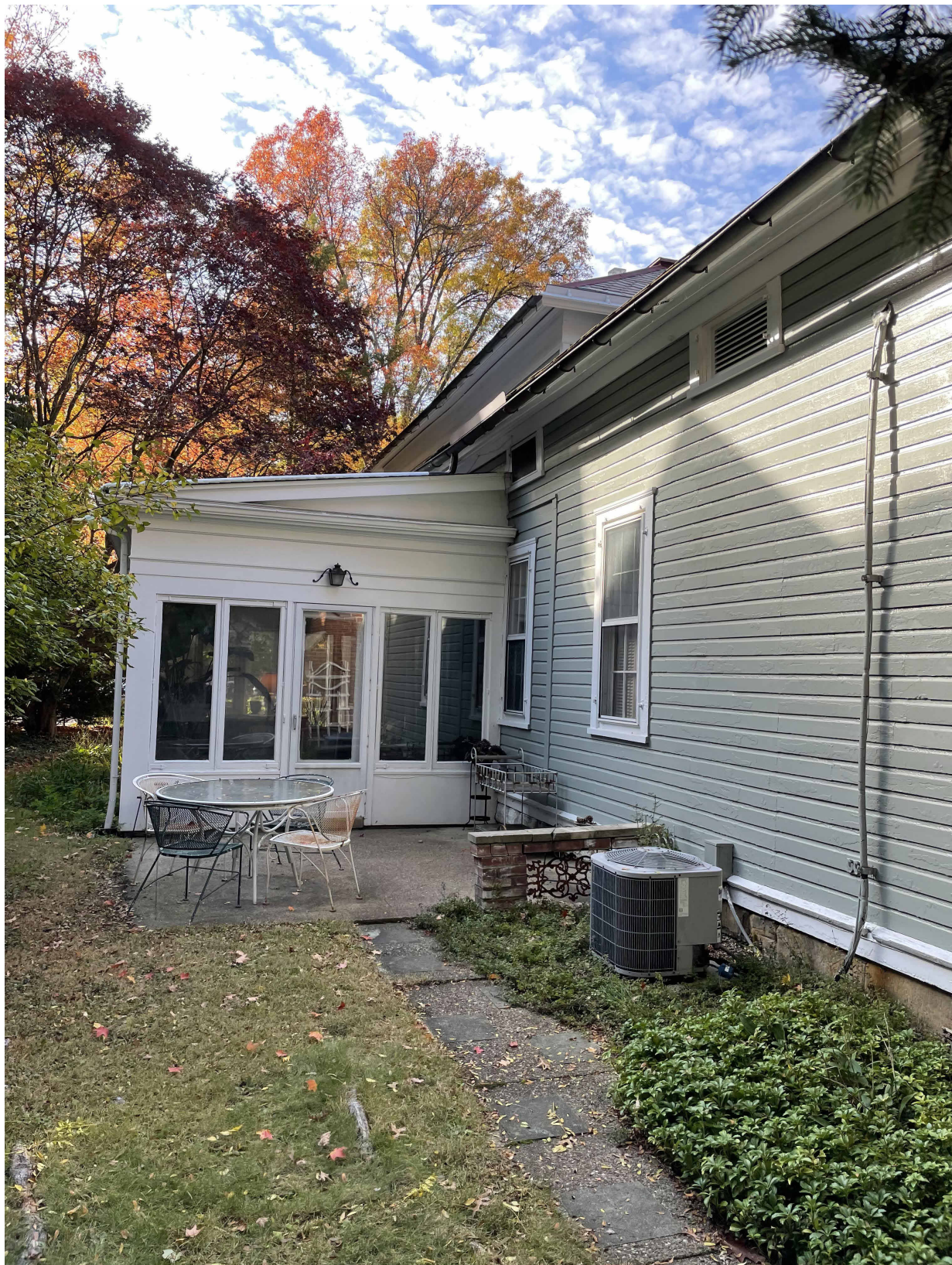
SOUTH ELEVATION - FROM BACK YARD
