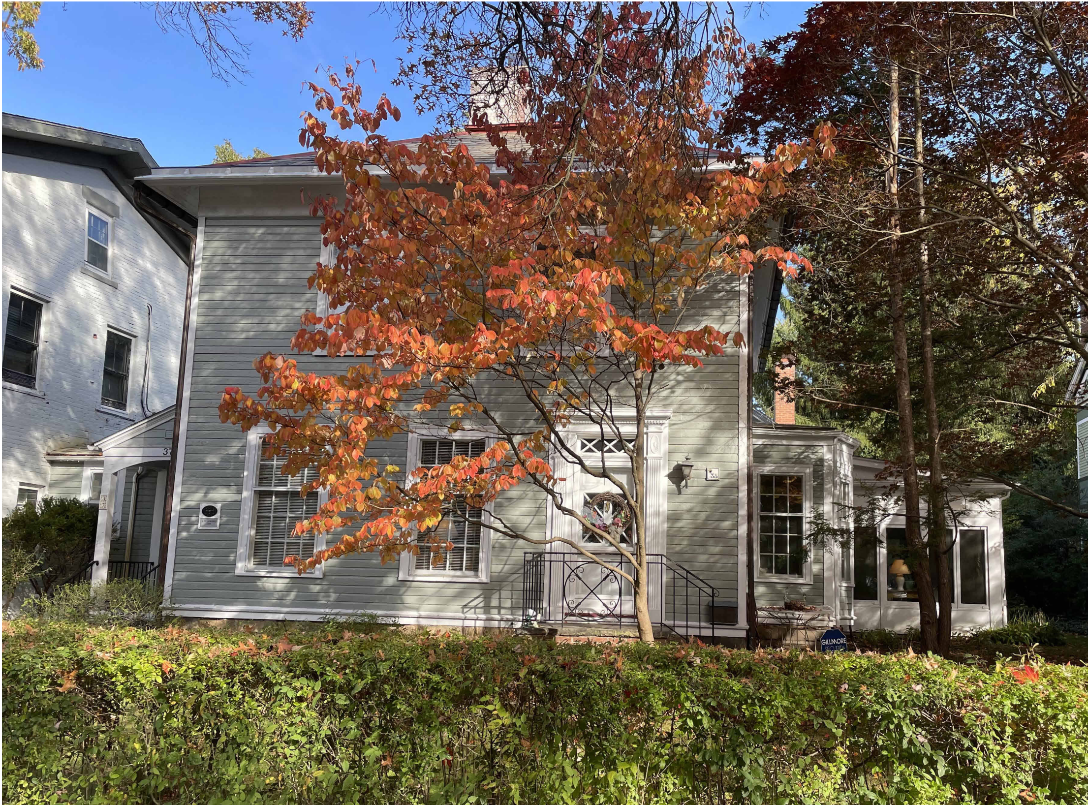
WEST ELEVATION - SHOWING SUN PORCH
