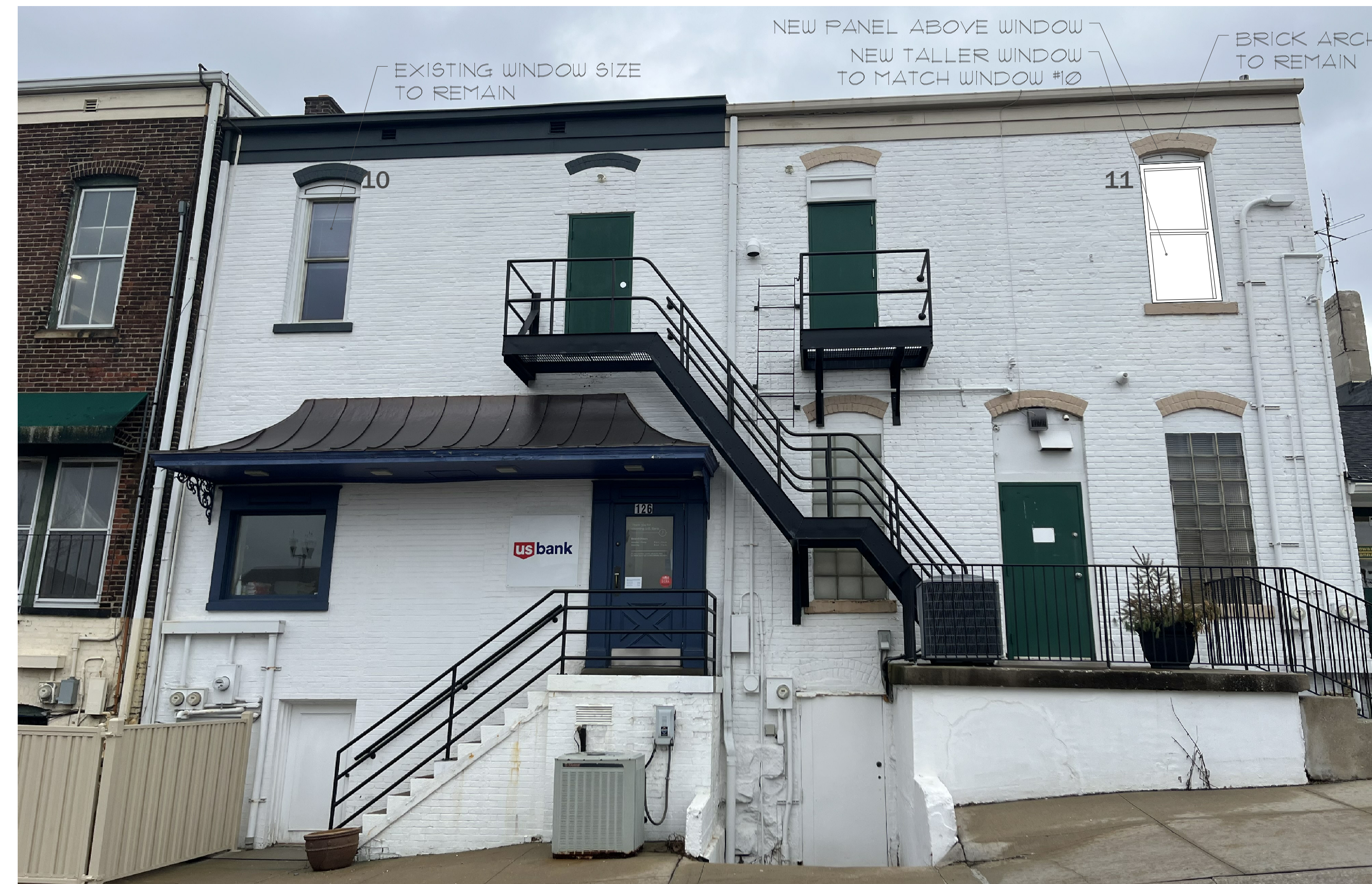
4 REAR ELEVATION - PROPOSED SCALE: 1/4" = 1'-0"
