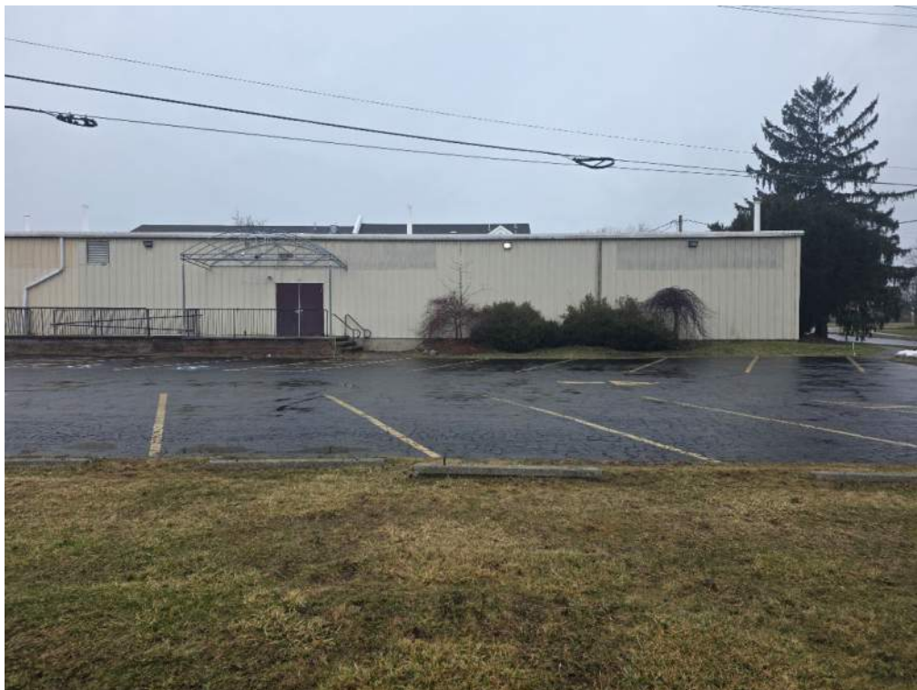
Photograph 6 View facing west depicting site conditions at Data Point 3 (non-wetland)
